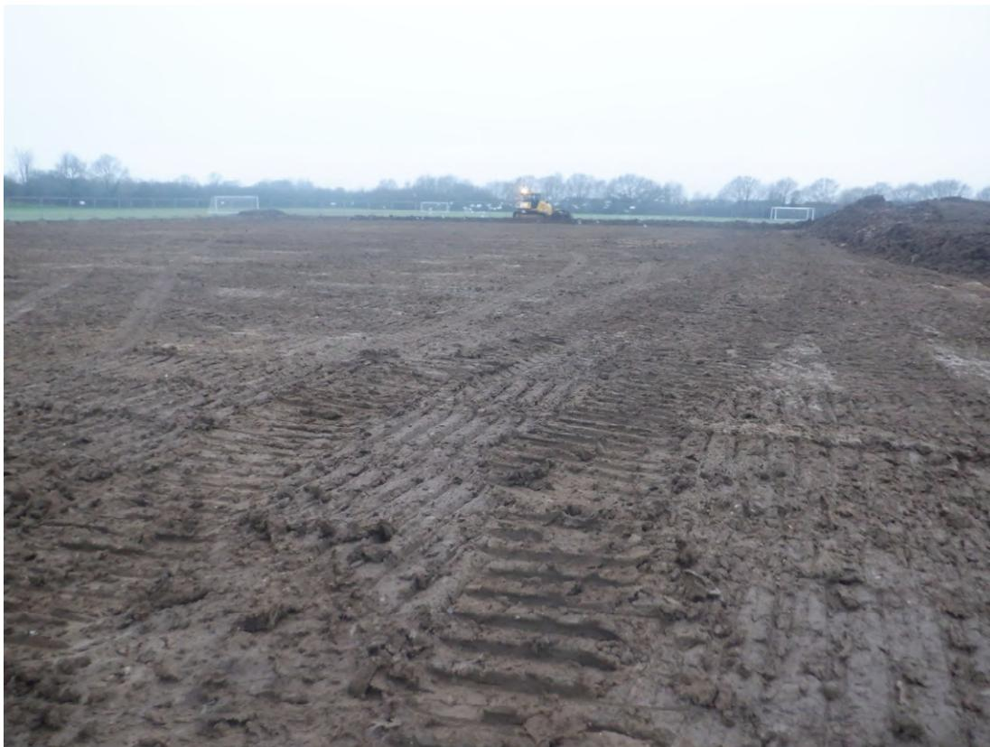
**Photograph 1** Strip of the sports pitch with a bulldozer, looking north-west.
