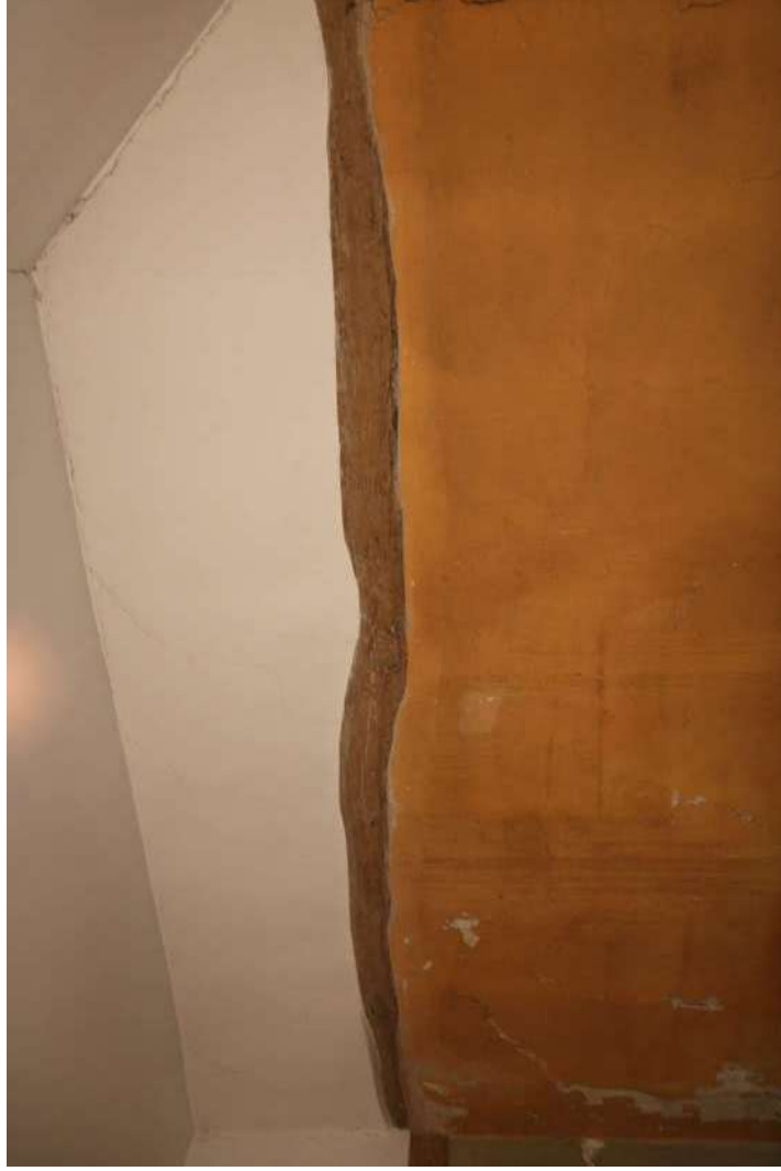
EEX60240_PhotoGraph_087 Detail of gable tie-beam in eastern wall of room 11. Photograph taken facing north-east.
