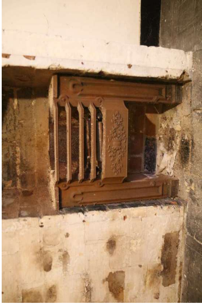
EEX60240_PhotoGraph_079 Detail of cast iron hob grate in fireplace of room 10. Photograph taken facing east.
