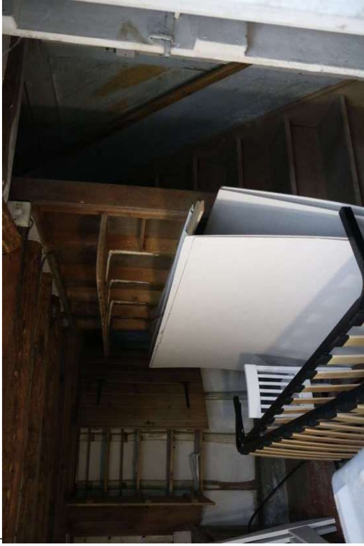
EEX60240_Phograph_050 Detail of three diagonal through bracing made from hand sewn timbers in room 5, facing east
