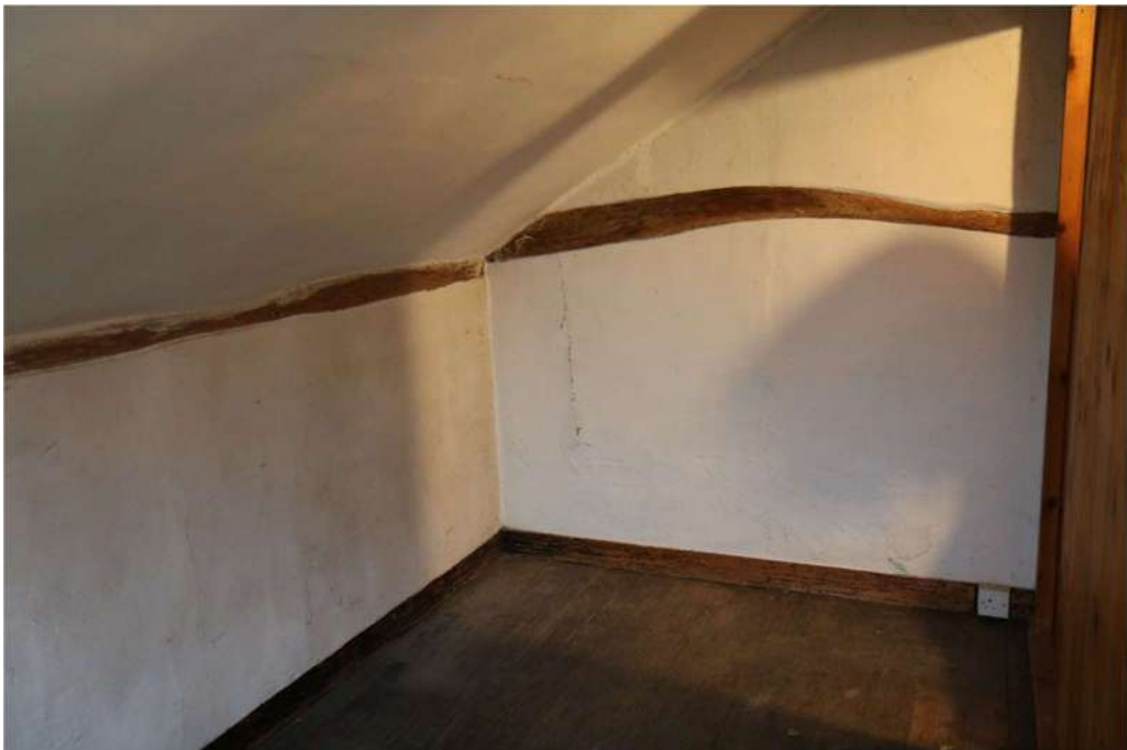
Photograph 14 Detail of exposed aisle tie-beam and wall-plate in room 8. Photograph taken facing north-east.
