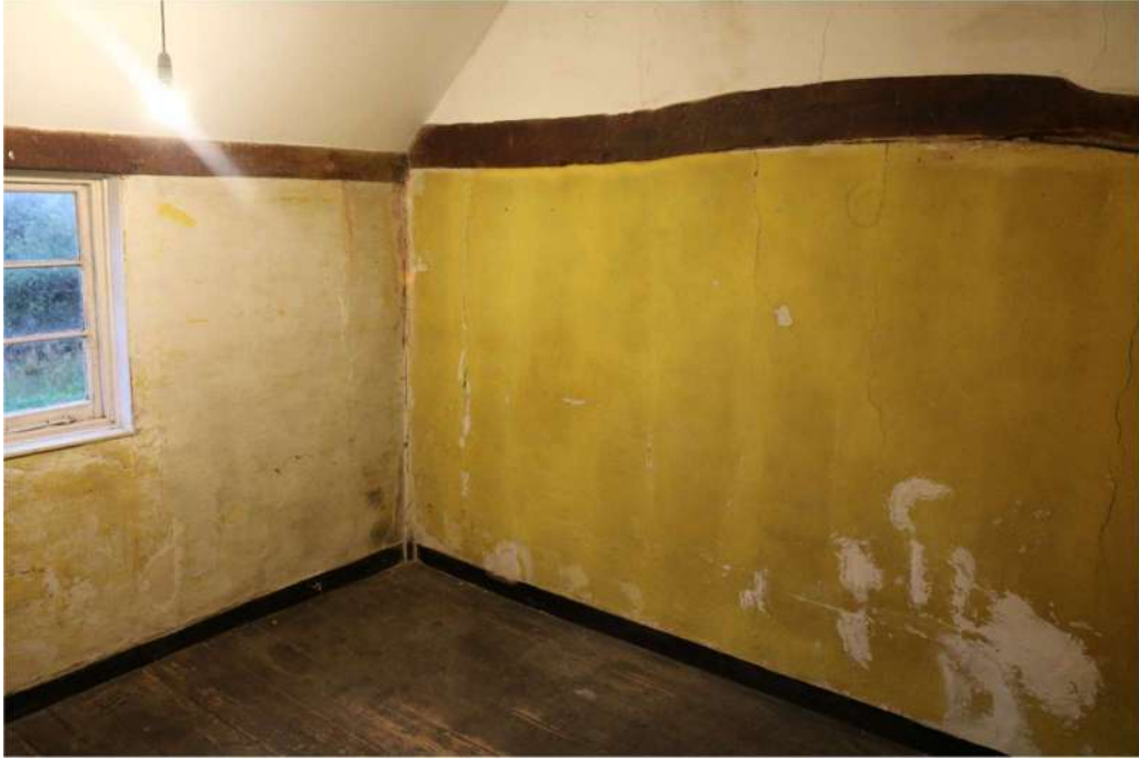
Photograph 16 Interior of room 10, evidence of hidden framing in yellow wall. Photograph taken facing south-west.
