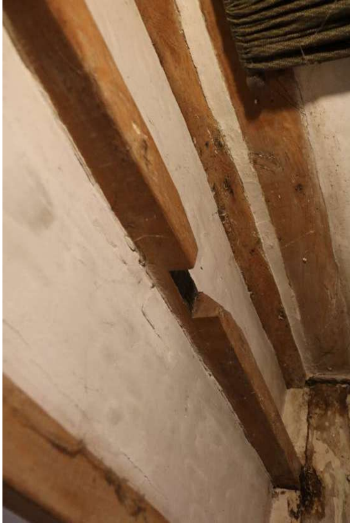
EEX60240_Phograph_035 Detail of reused joist in ceiling of room 2. Photograph taken facing south-east.
