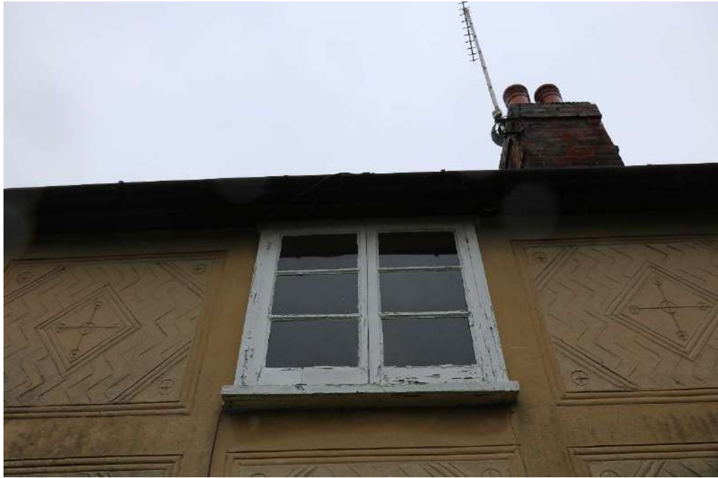
Photograph 2 Detail of window on first floor of southern elevation, with imitation pargeting either side. Photograph taken facing north.
