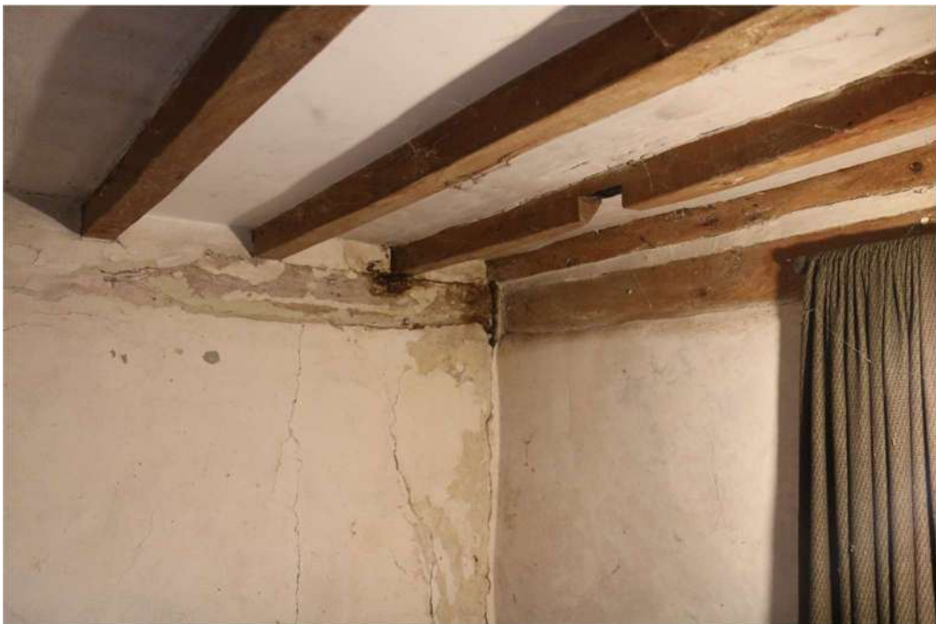
Photograph 10 Detail of exposed girding beams and reused joist in room 2. Photograph taken facing south-east.
