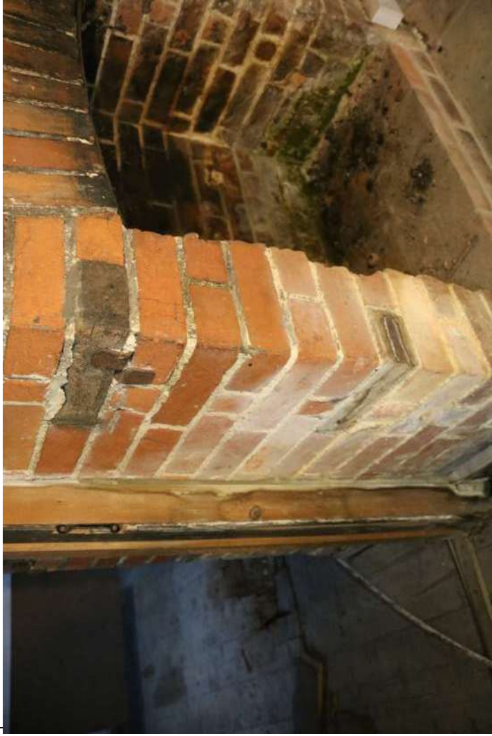
EEX60240_Phograph_038 Timber nogs in fireplace located in room 2. Photograph taken facing north-west.
