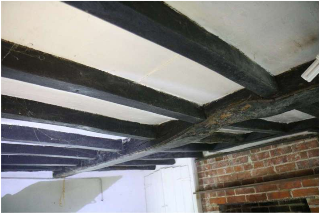
Photograph 8 Detail of joists and binding beam in ceiling of room 1. Photograph taken facing north north-east.
