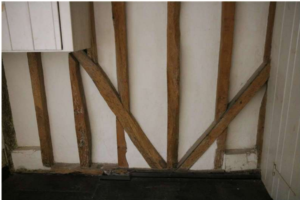
Photograph 15 Detail of diagonal through-bracing on southern wall in room 9. Photograph taken facing south.
