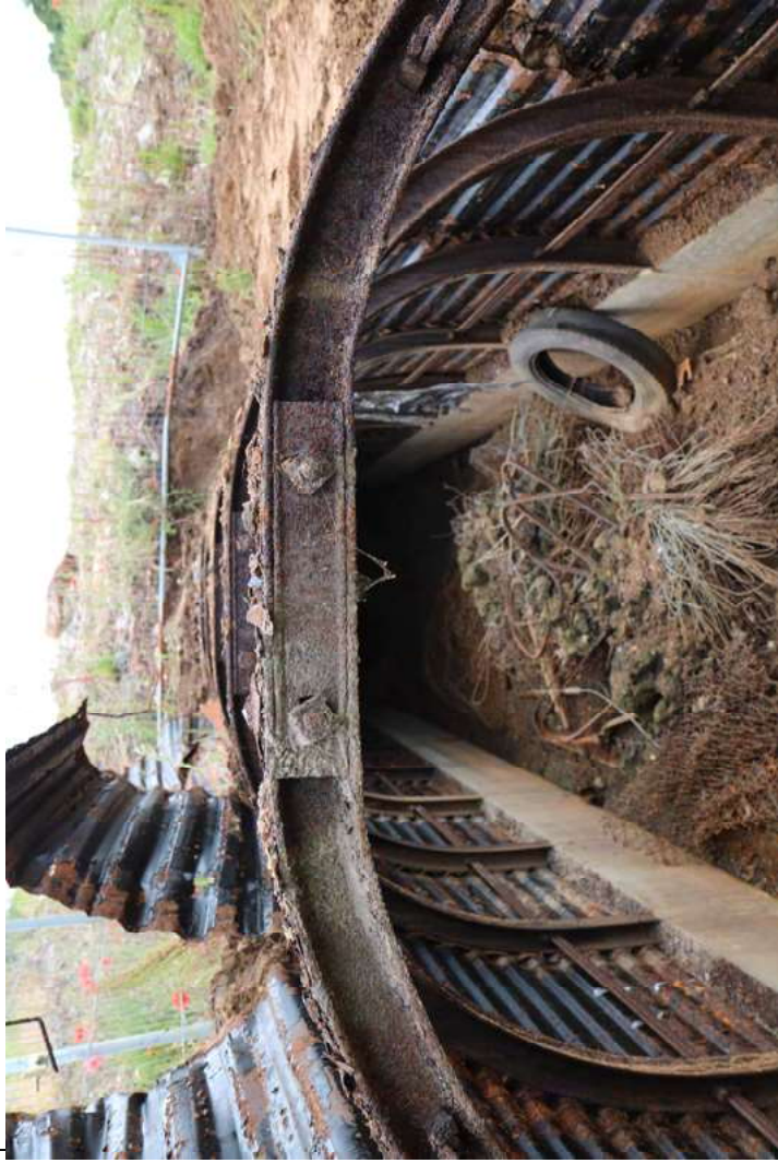
2024.05c_Photograph_006 Detail of fishplate and square-headed bolts in frame of shelter one. Photograph taken facing south-east.
