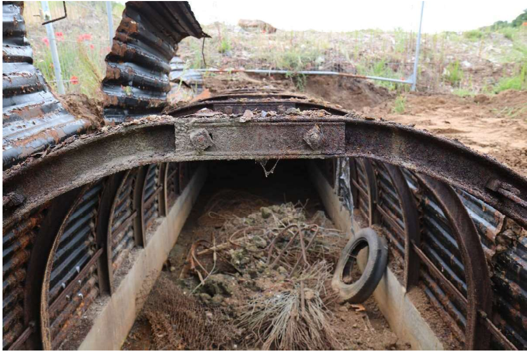
Photograph 3 Detail of fish-plate and square-headed bolts in frame of shelter one. Photograph taken facing south-east.
