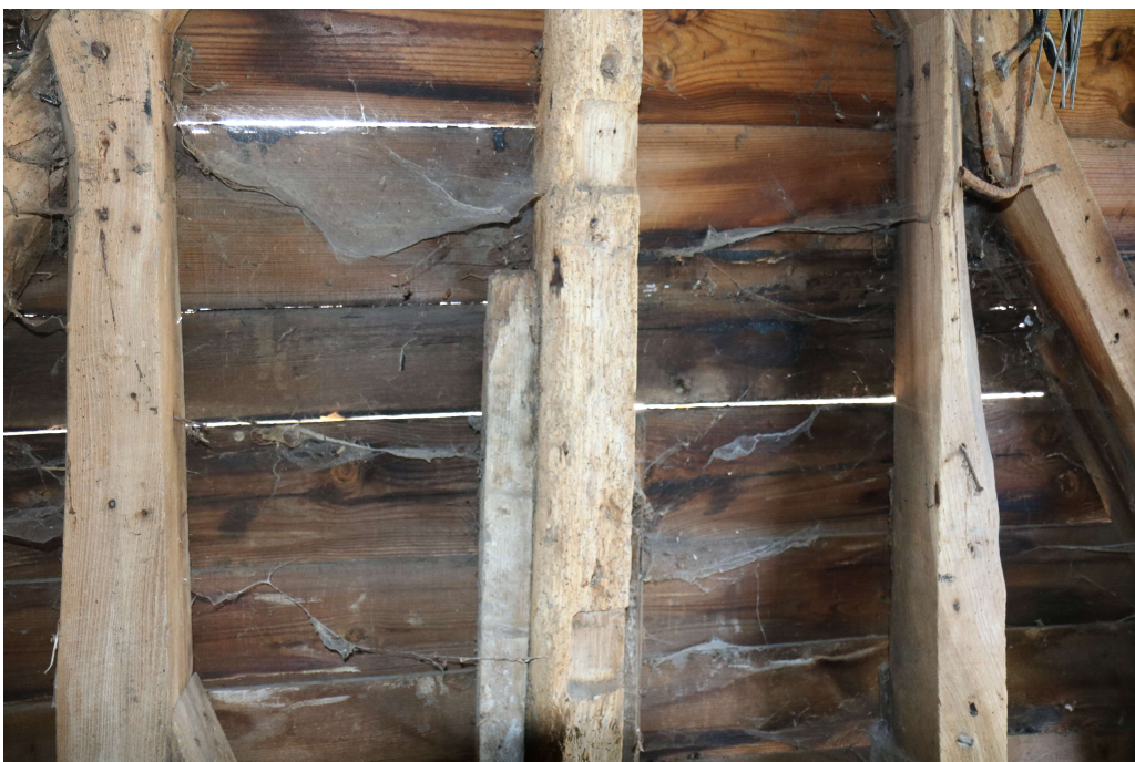
Photograph 15 Detail of re-used timbers in barn, Bay 1. Photograph taken facing south-east.
