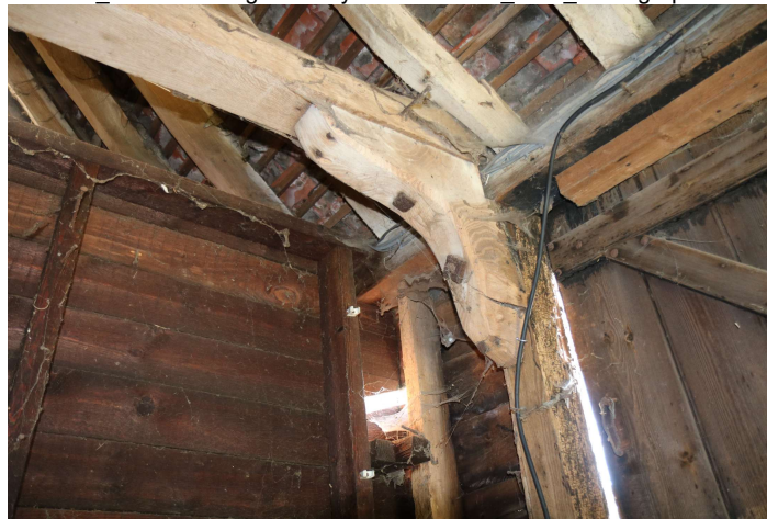
WHGB23_PhotoGraph_0047 Detail of knee-brace in barn, bay 1. Photogra...
