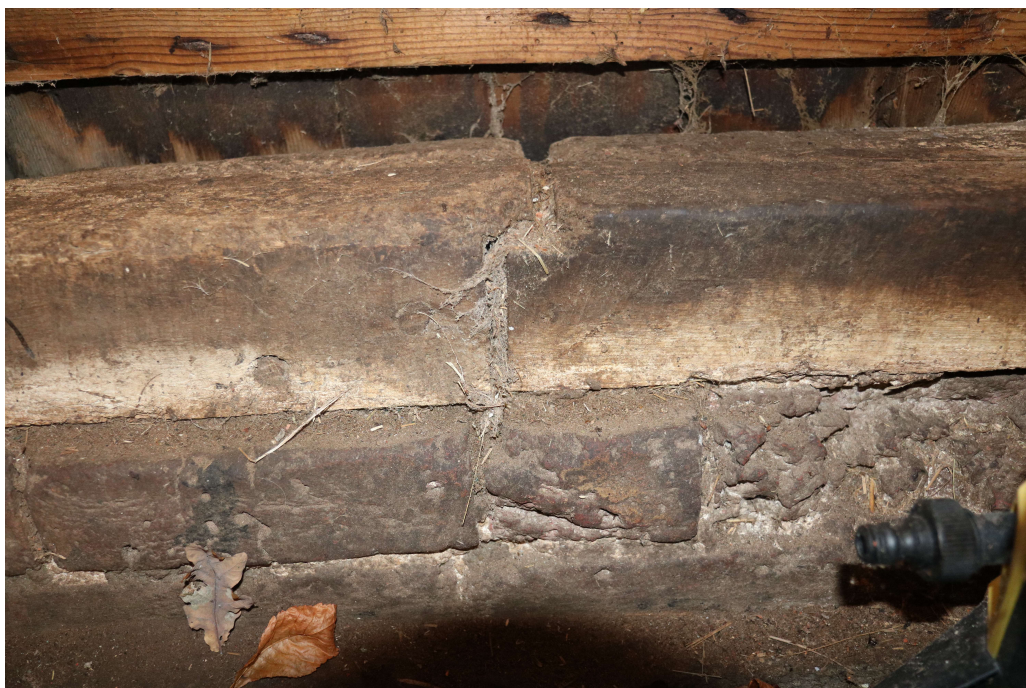
Photograph 16 Detail of scarf-joint on sill-beam beneath northern doorway in barn, Bay 2. Photograph taken facing north/north-west.
