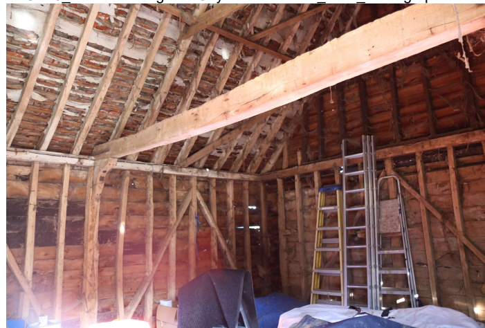
WHGB23_PhotoGraph_0065 Detail of tie-beam between bays 2 and 3 of b...
