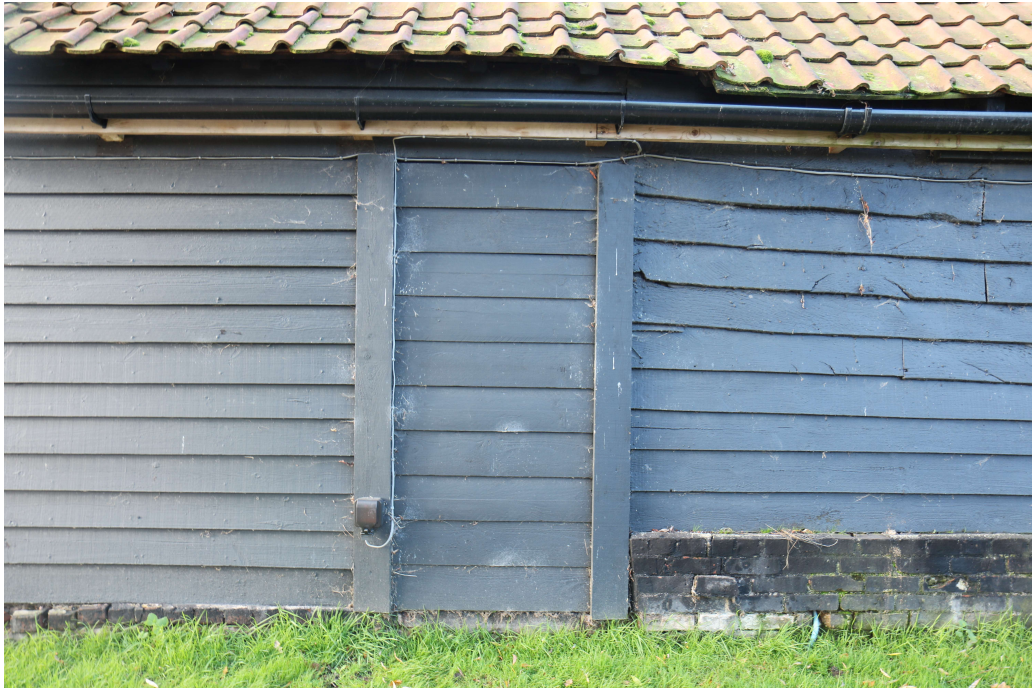
Photograph 31 Detail of blocked doorway on north-east elevation. Photograph taken facing south-west.
