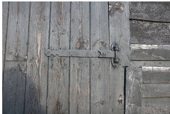
WHGB23_PhotoGraph_0014 Detail of strap hinge on barn door (south-east...
