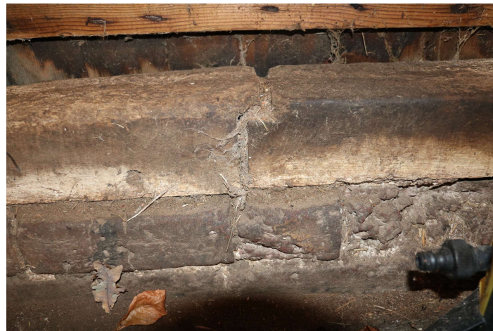
WHGB23_PhotoGraph_0071 Detail of scarf joint on sill beam beneath nort...
