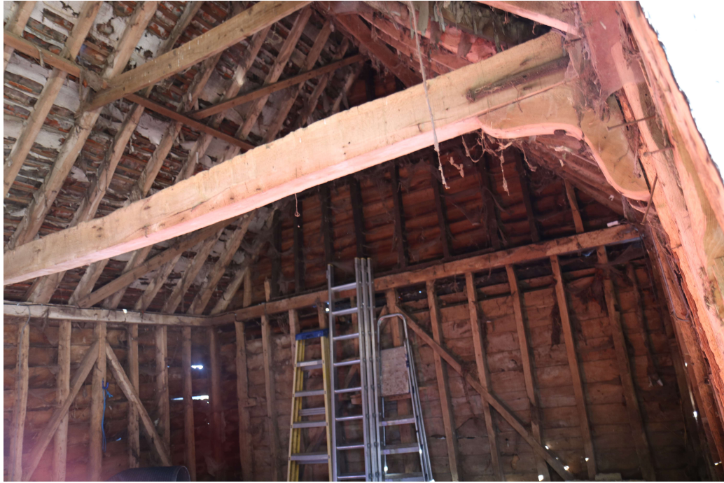
Photograph 8 Detail of knee-brace and roof construction in barn, Bay 2. Photograph taken facing north-east.
