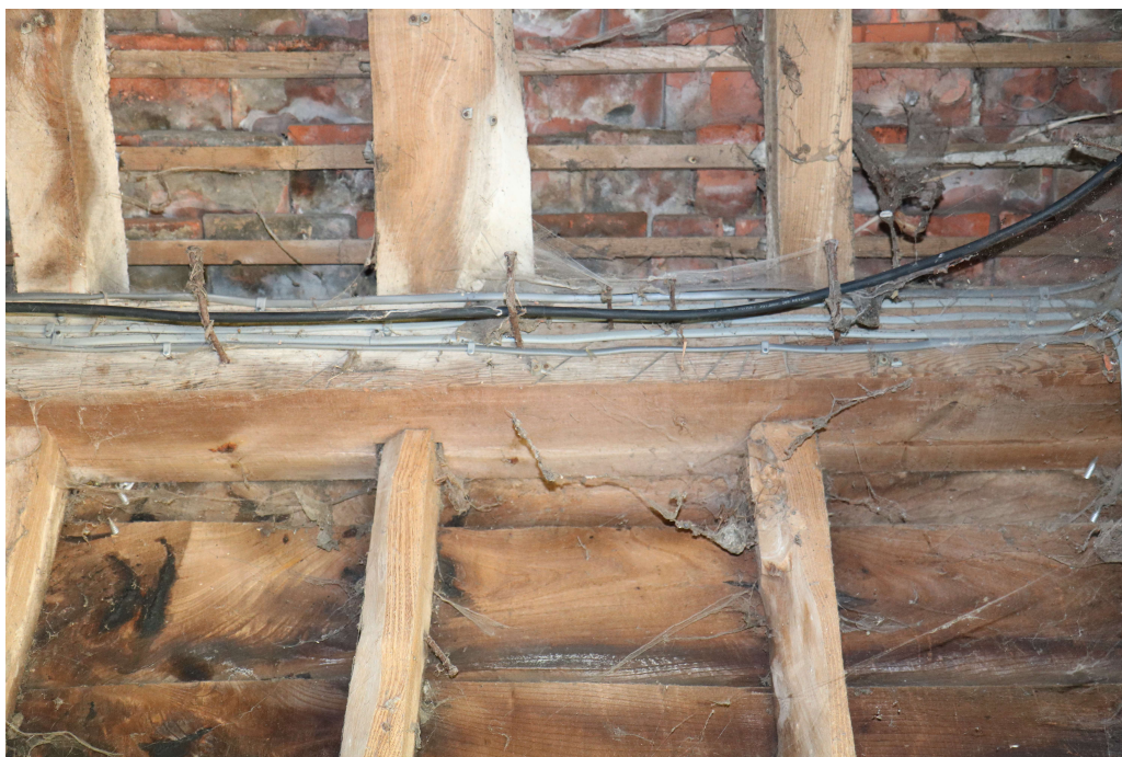
Photograph 14 Detail of Baltic timber mark on wall plate in barn, Bay 1. Photograph taken facing south-east.
