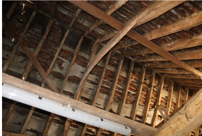
WHGB23_PhotoGraph_0050 Detail of tie-beam and roof construction of ba...
