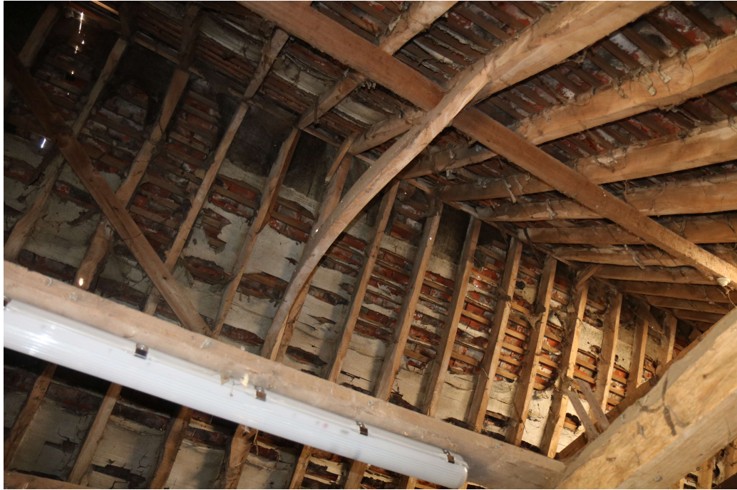
Photograph 10 Detail of Tie Beam and roof construction of barn, Bay 1. Photograph taken facing north.
