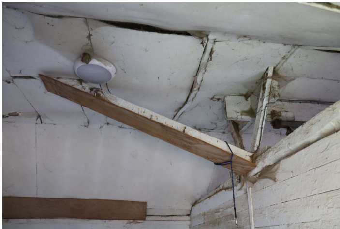
WHGB23_PhotoGraph_0037 Detail of inclined strut in stable 1. Photograph...
