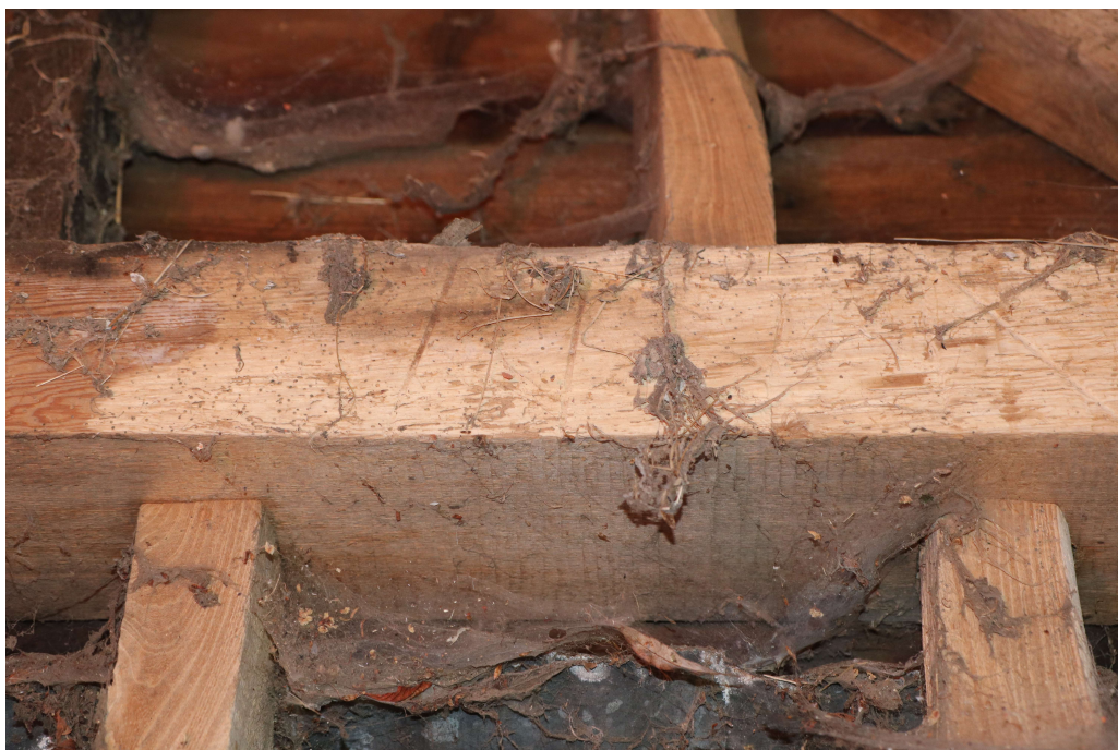
Photograph 22 Detail of Baltic timber mark on north-eastern wall-plate in barn, Bay 3. Photograph taken facing north-east.
