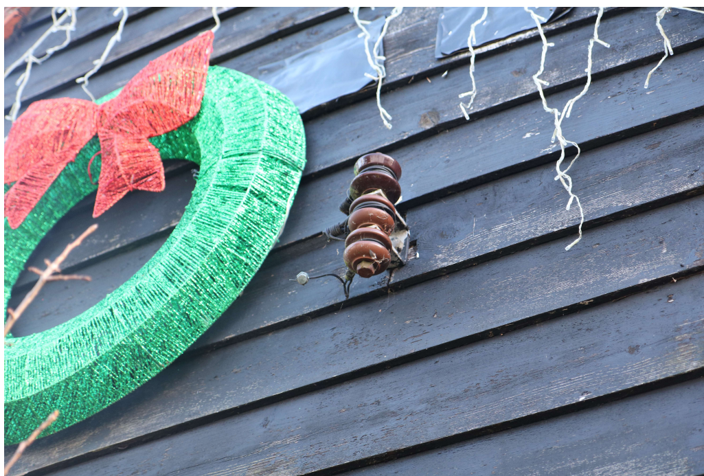
Photograph 5 Detail of ceramic electricity point port on south-west elevation. Photograph taken facing north-east.
