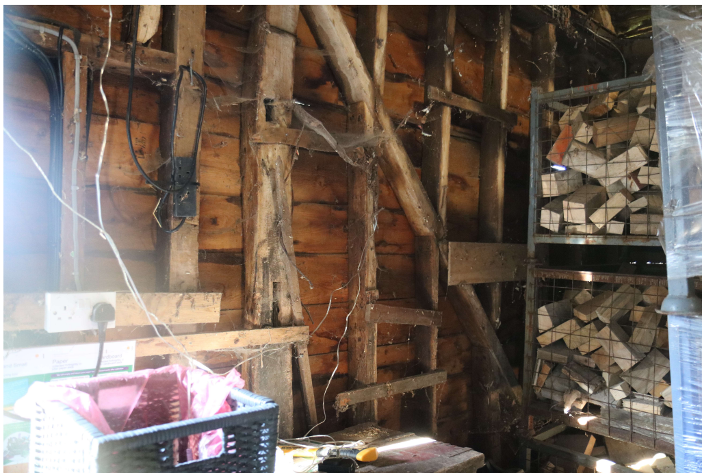
Photograph 12 Detail of re-used timbers and timber frame construction in barn, Bay 1. Photograph taken facing west.
