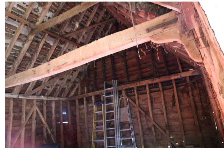
WHGB23_PhotoGraph_0066 Detail of knee-brace and roof construction in ...
