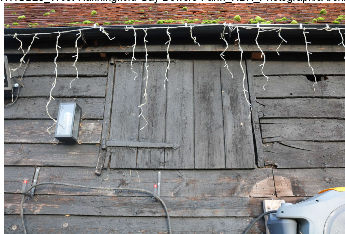
WHGB23_PhotoGraph_0011 Detail of pitching door on south-eastern eleva...
