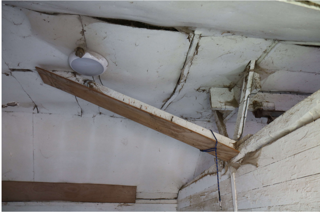
Photograph 35 Detail of inclined strut in stable 1. Photograph taken facing north-east.
