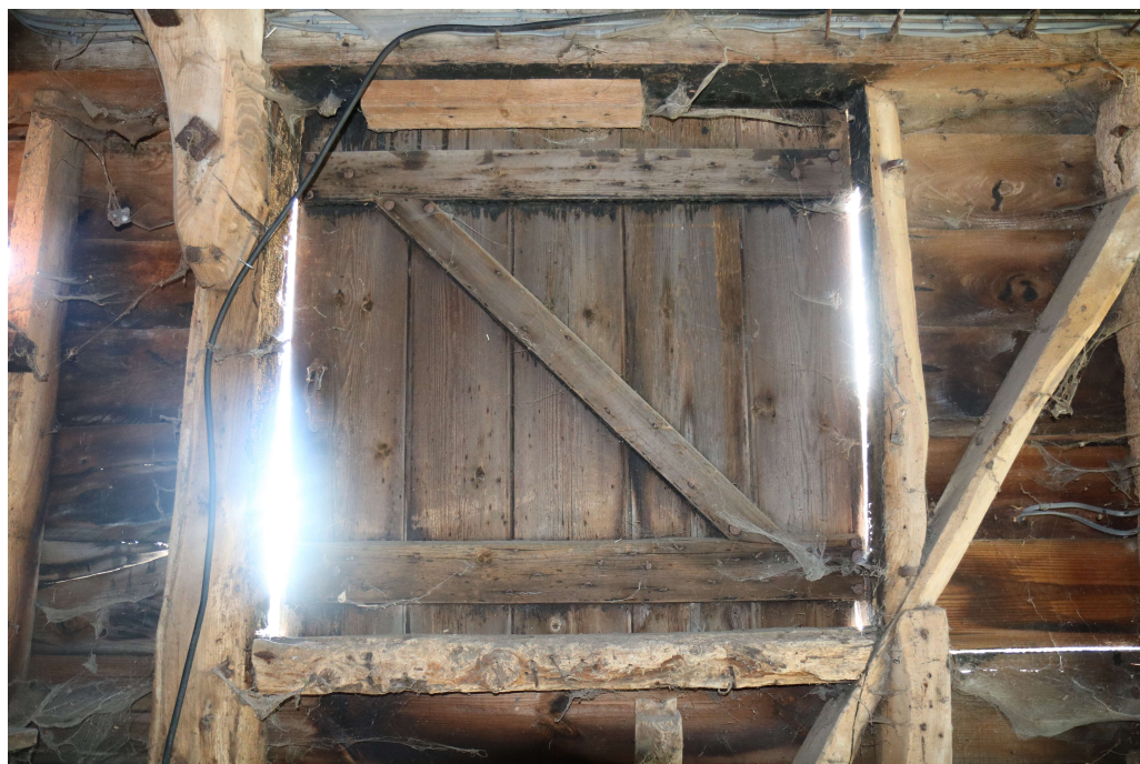
Photograph 13 Detail of pitching door in barn, Bay 1. Photograph taken facing south-east.
