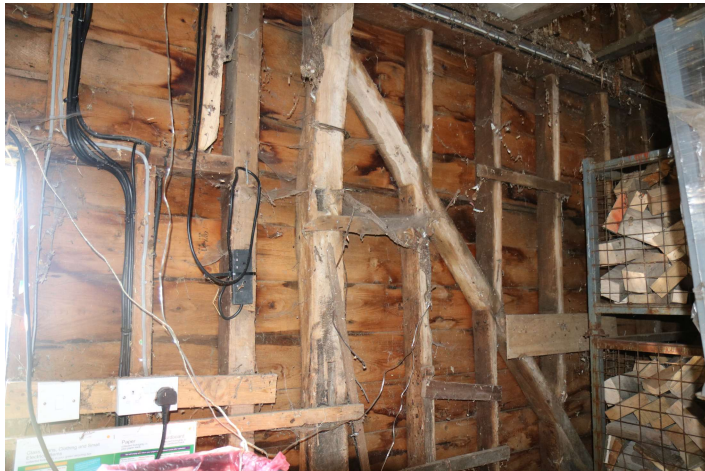
WHGB23_PhotoGraph_0052 Detail of re-used timber in barn, bay 1. Photo...
