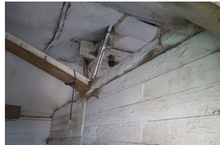
WHGB23_PhotoGraph_0039 Detail of tie-beam between stable 1 and 2. P...
