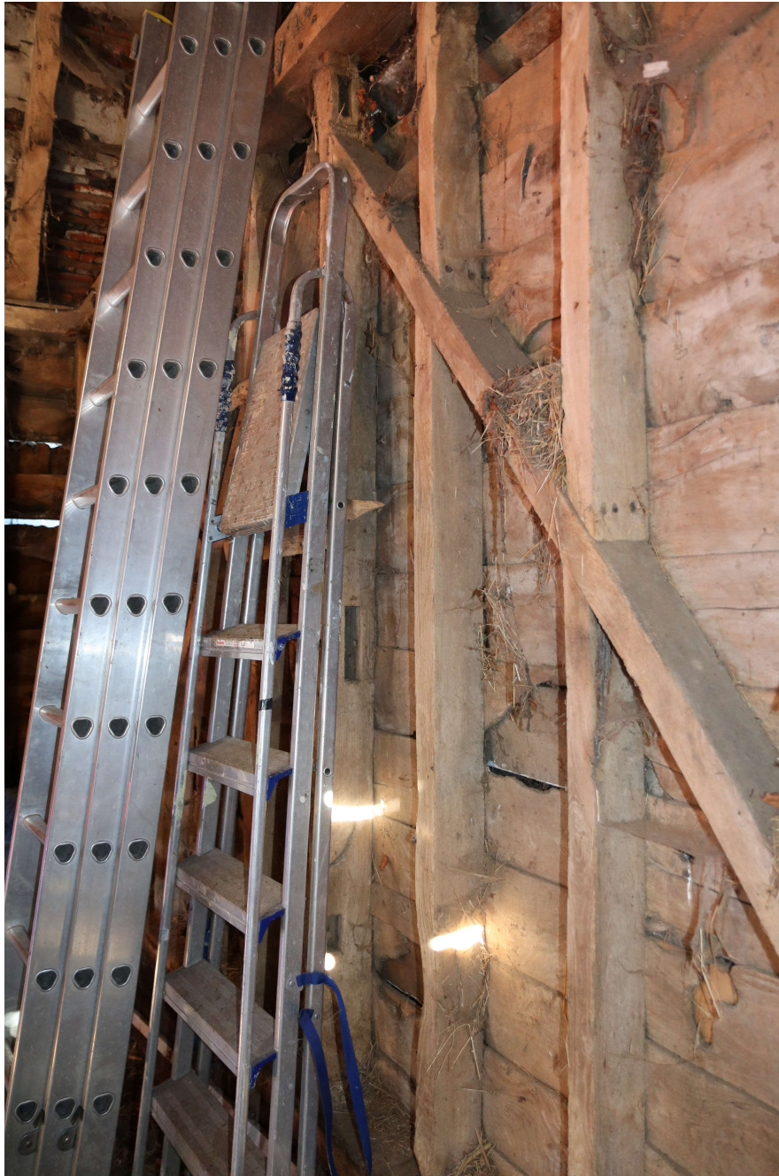
Photograph 26 Detail of re-used stud in north-eastern wall of barn, Bay 3. Photograph taken facing north.
