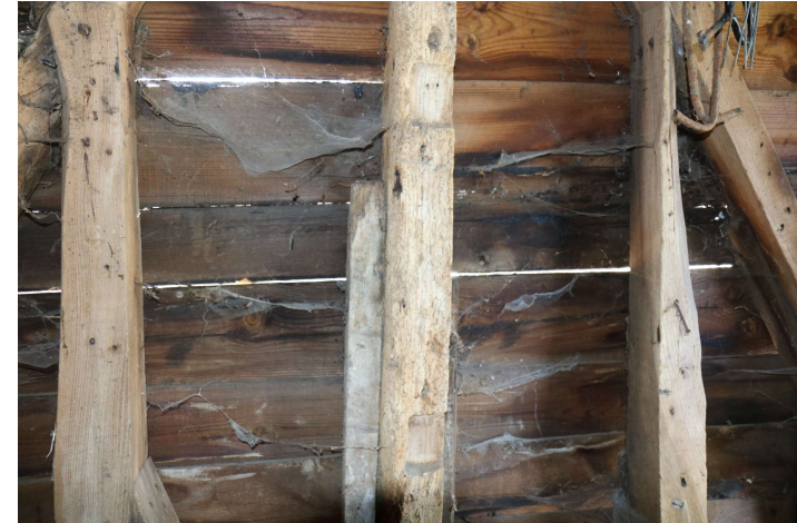
WHGB23_PhotoGraph_0051 Detail of re-used timbers in barn, bay 1. Phot...
