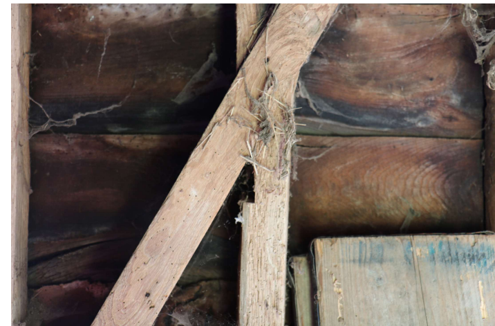
WHGB23_PhotoGraph_0072 Detail of re-used stud in south-eastern wall of...
