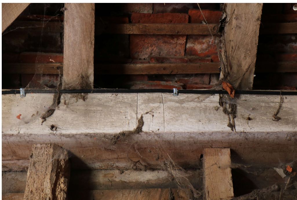
Photograph 23 Detail of Baltic timber mark on north-western wall-plate in barn, Bay 3. Photograph taken facing north-west.
