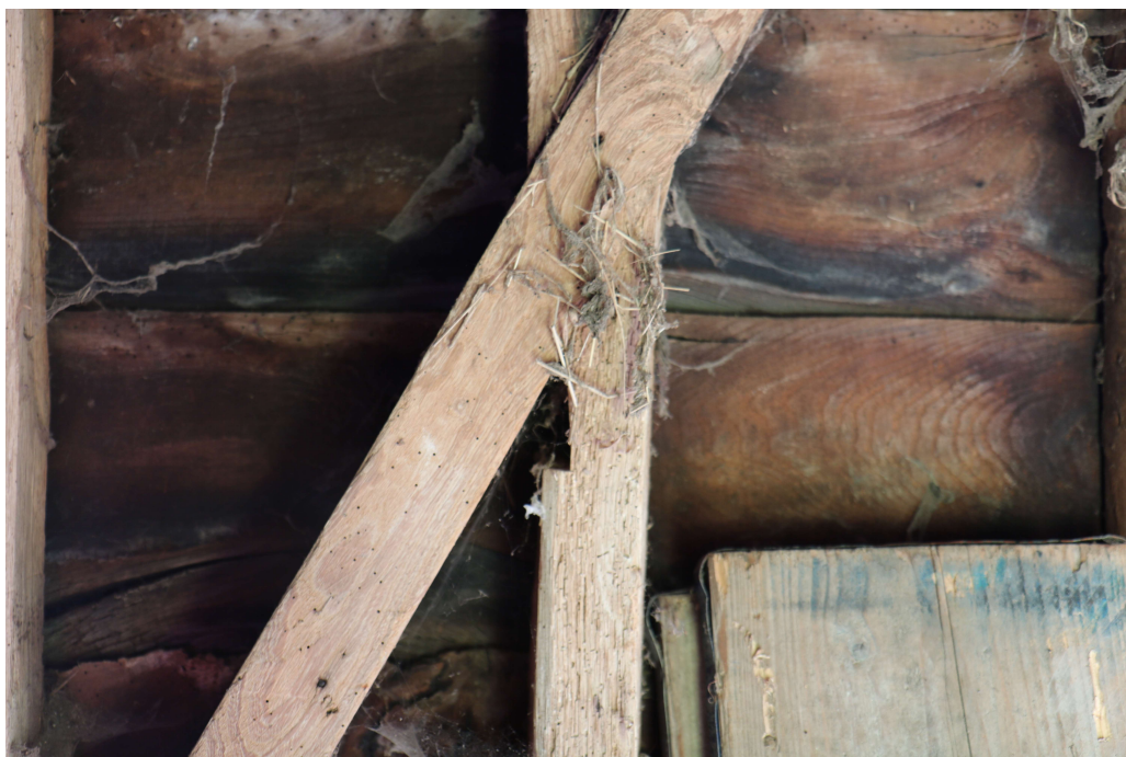
Photograph 18 Detail of re-used stud in south-eastern wall of barn, Bay 2. Photograph taken facing south/south-east.
