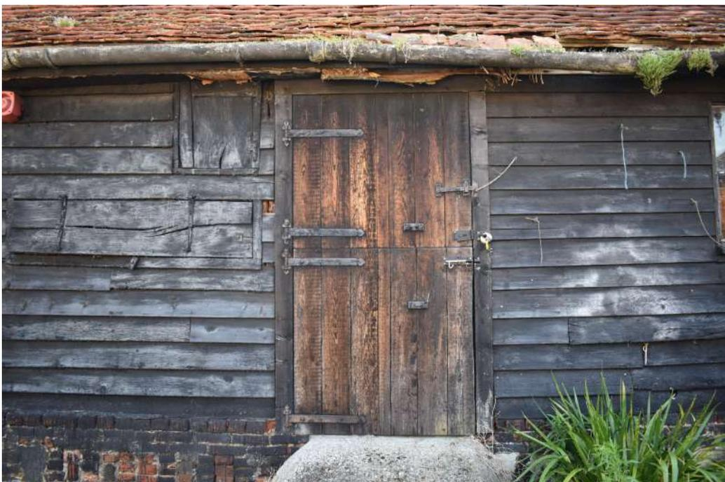
**Photograph 3** Detail of doors and hatch on western elevation, showing charred weatherboard. Photograph taken facing east.
