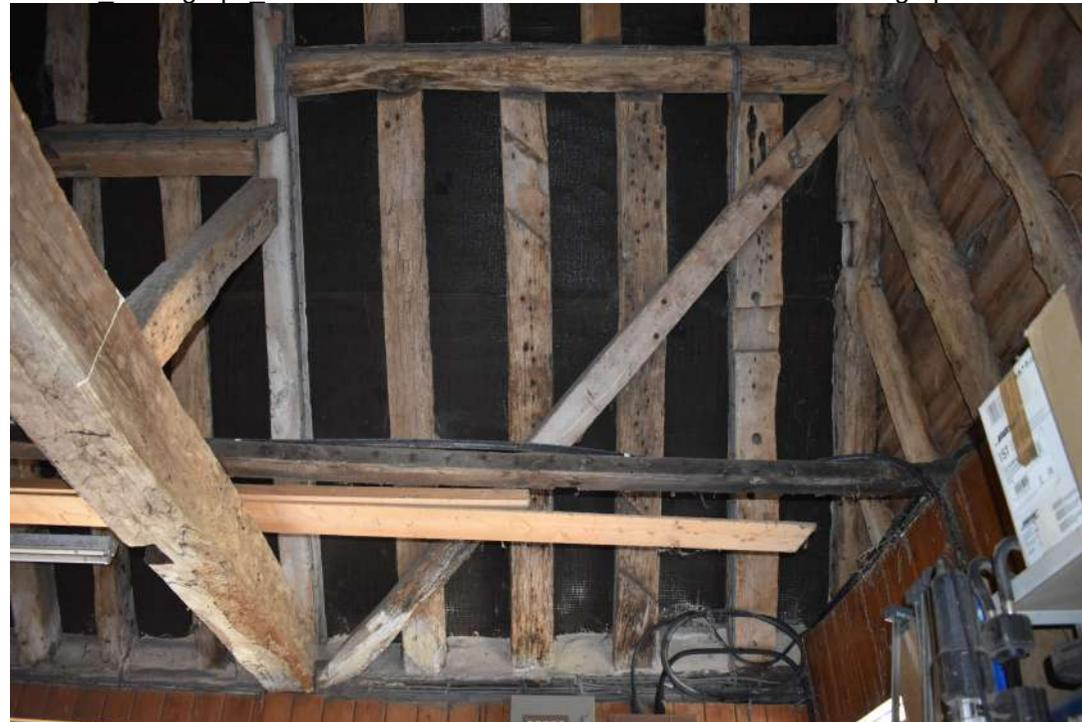
LBGG23\_Photograph\_036Detail of roof structure showing reused rafters in western roof pit...
