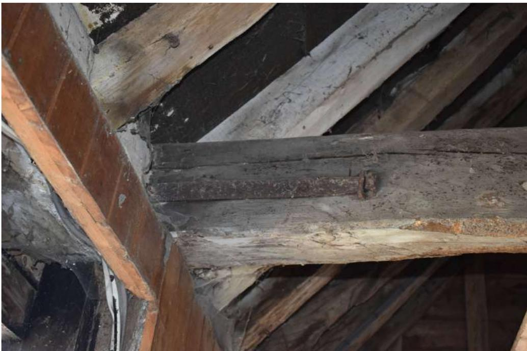
**Photograph 11** Detail of tie-beam strap between bays 1 and 2 of stable 1. Photograph taken facing north.
