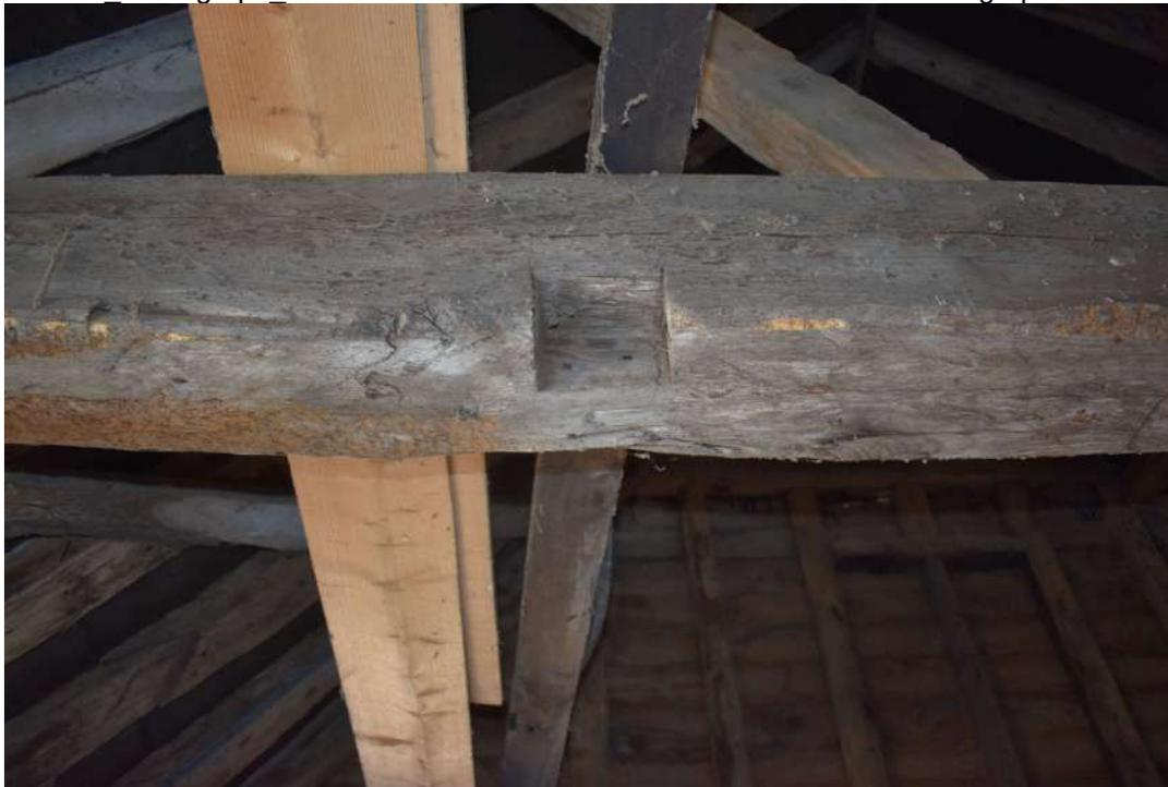
LBGG23\_Photograph\_035Detail of reused tie-beam in bay 1 of stable 1. Photograph taken from...
