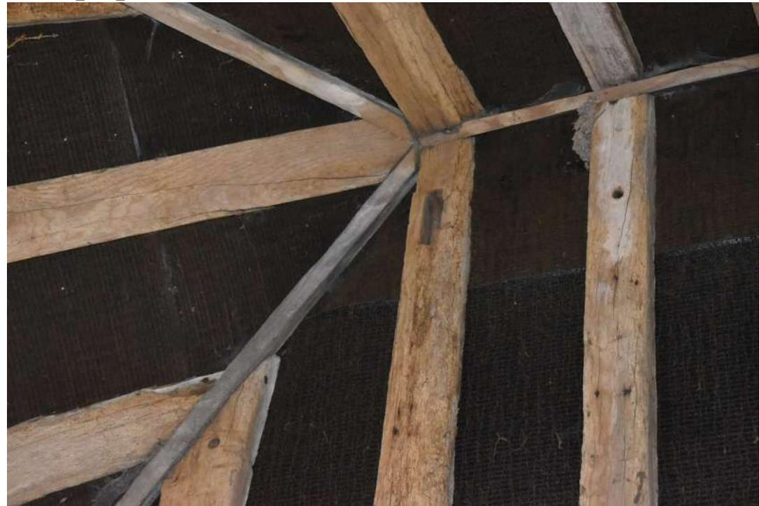
LBGG23 Photograph\_041Detail of tie-beam strap between bays 1 and 2 of stable 1. Photog... LBGG23 Photograph\_042Detail of reused rafter in eastern roof pitch of bay 1 of stable 1. P...
