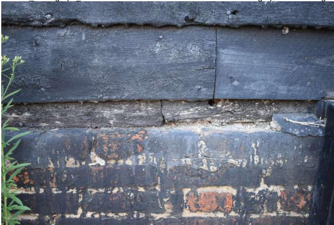
LBGG23\_Photograph\_019Detail of ?scarf-joint in western sill-beam. Photograph taken facin...
