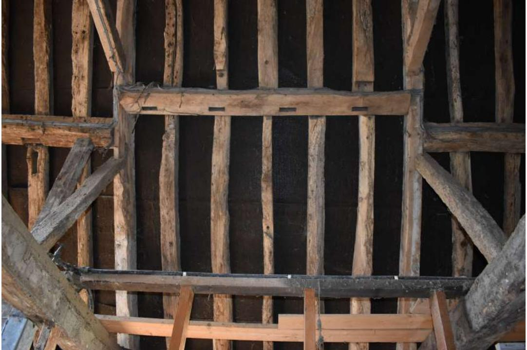
LBGG23\_Photograph\_055Detail of roof structure, showing reused timbers, of eastern roof p...
