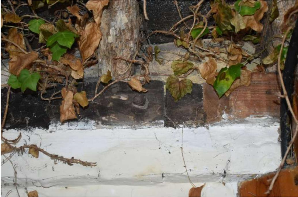
**Photograph 15** Detail of scarf-joint in eastern wall-plate in bay 3 of stable 1.
