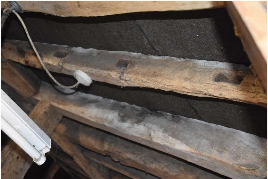
LBGG23 Photograph\_045Detail of reused tie-beam with iron strap, between bays 2 and 3 o...
