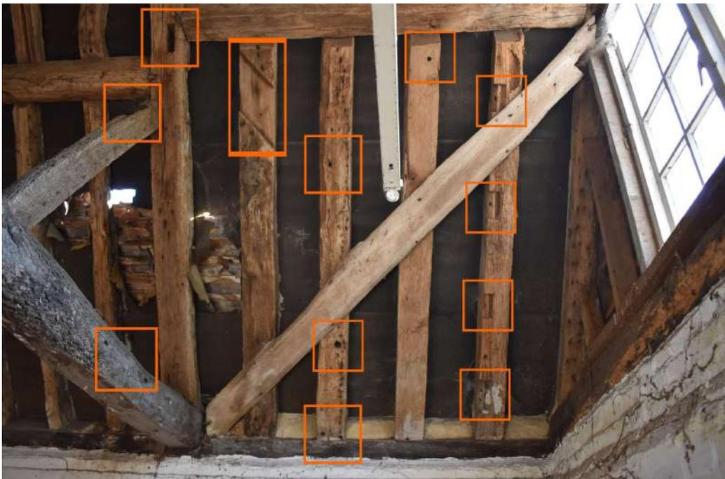
**Photograph 18** Detail of roof structure of eastern roof pitch of bay 7 of stable 1. Evidence of reused highlighted in orange. Photograph taken facing east.
