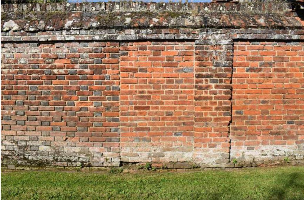
**Photograph 8** Detail of blocked opening in wall, showing differences in bricks. Photograph taken facing west.
