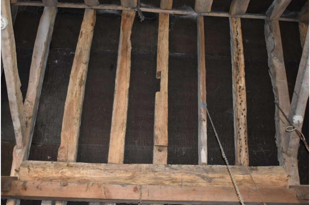
LBGG23\_Photograph\_047Detail of scarf-joint in eastern wall-plate in bay 3 of stable 1. Phot...
