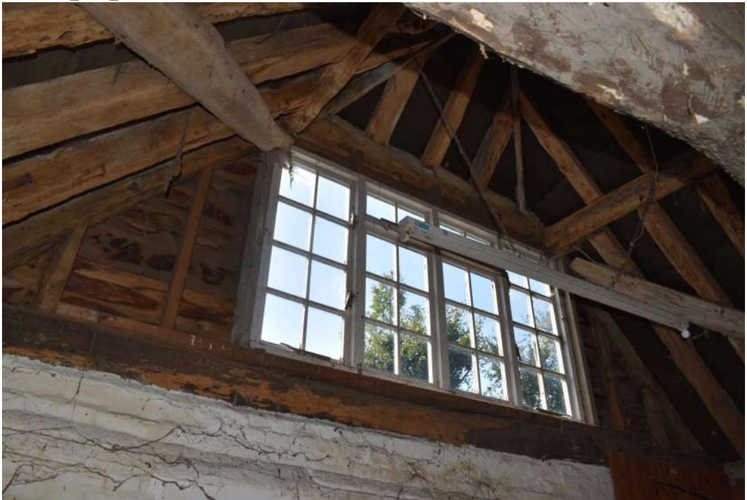
LBGG23 Photograph\_061Detail of roof structure, showing reused timbers, of western roof p...
