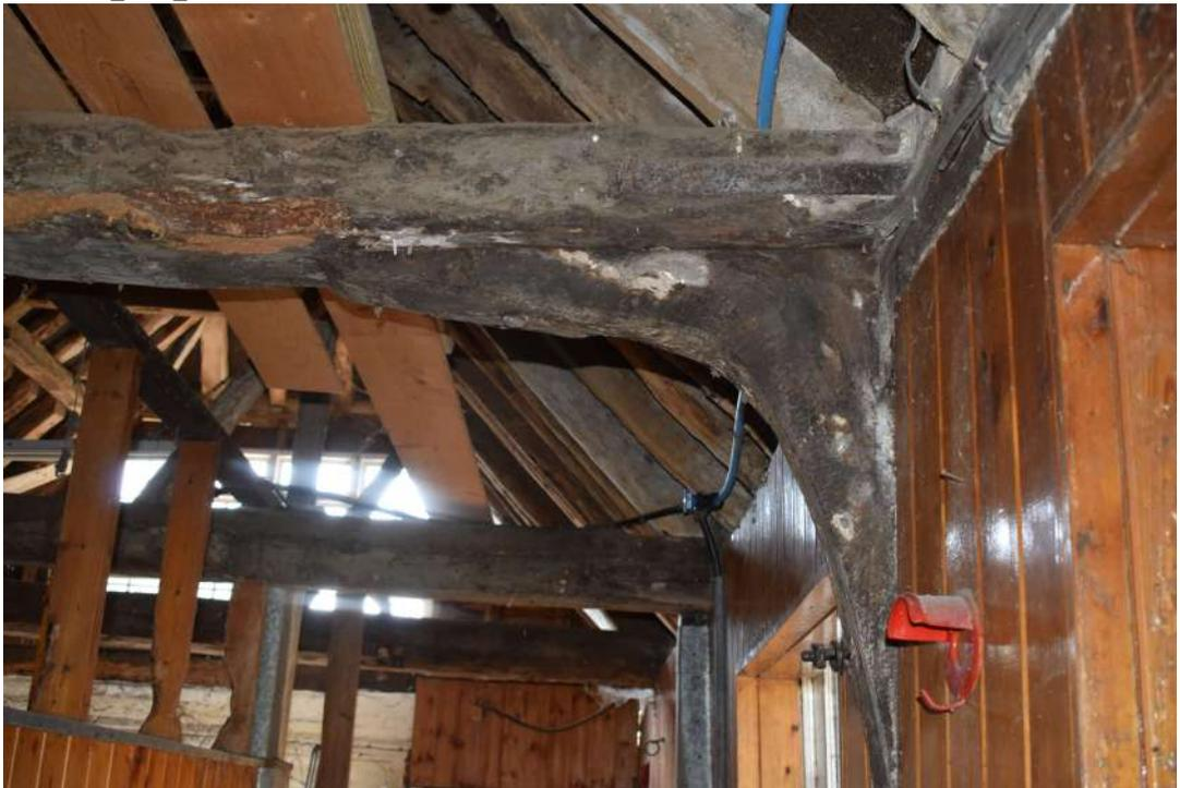
LBGG23 Photograph\_053Detail of roof structure, showing reused timbers, of western roof p...
