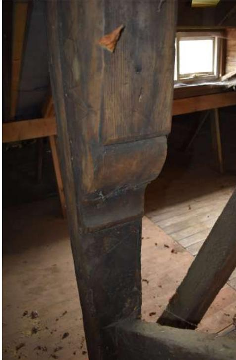
RHTHF23\_PhotoGraph\_123Detail of empty mortices from stud rem...
