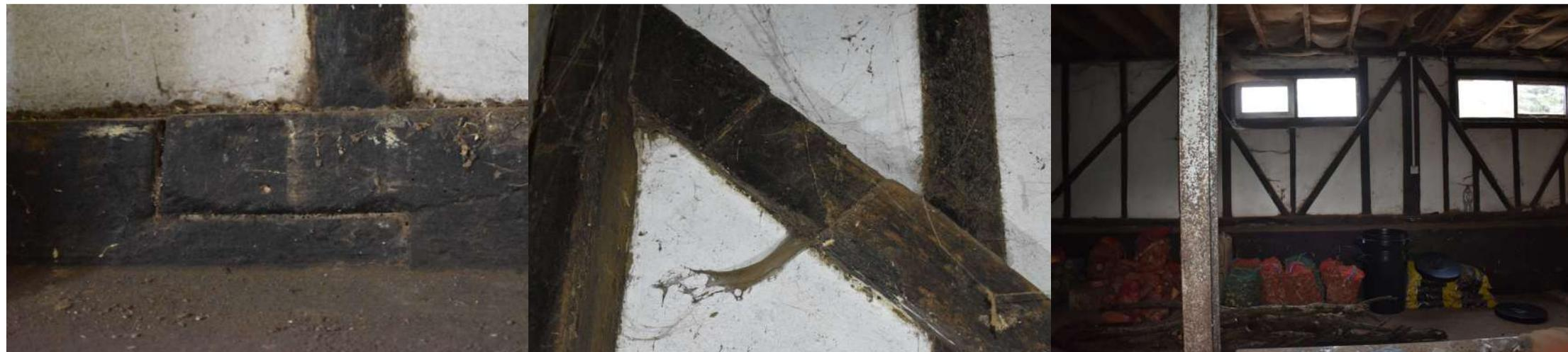
RHTHF23\_PhotoGraph\_145Detail of side-halved scarf joint in east... RHTHF23\_PhotoGraph\_146Detail of side-halved scarf joint in east... RHTHF23\_PhotoGraph\_147Detail of reused post in bay 3 of barn. ...
