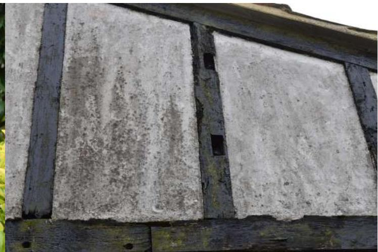
RHTHF23\_PhotoGraph\_052Detail of reused timbers and carpenter...
