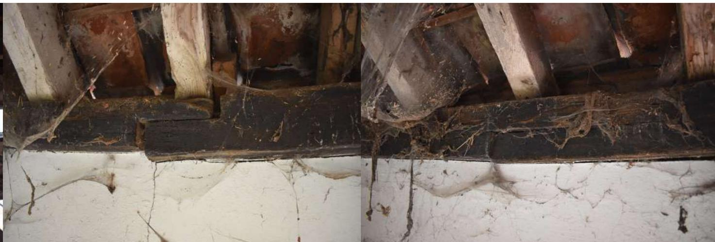
RHTHF23\_PhotoGraph\_106Detail of ?Baltic timber mark on corbel ... RHTHF23\_PhotoGraph\_107Detail of side-halved scarf joint in east... RHTHF23\_PhotoGraph\_108Eastern wall of bay 4 of barn, first floor....
