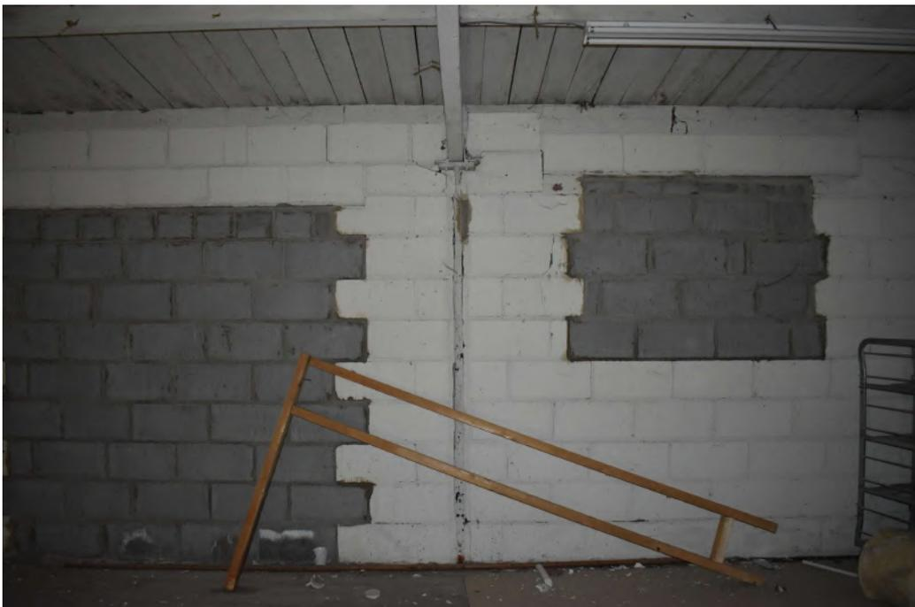
**Photograph 11** Detail of iron post in south-west wall of outbuilding 2. Photograph taken facing south-west.
