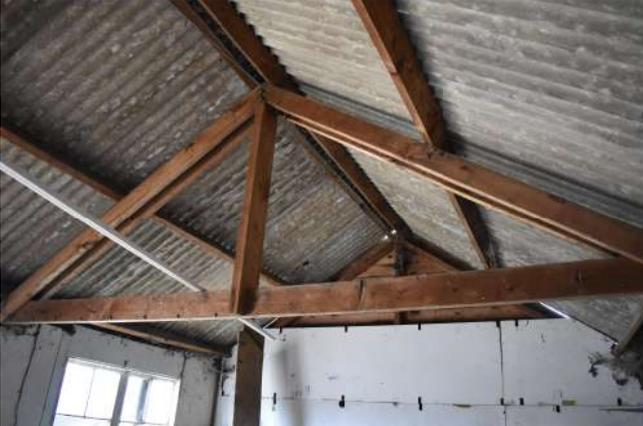
GEAGE23\_PhotoGraph\_049.JPG Detail of truss in sectional timber hut. Photograph taken facing north-w est.
