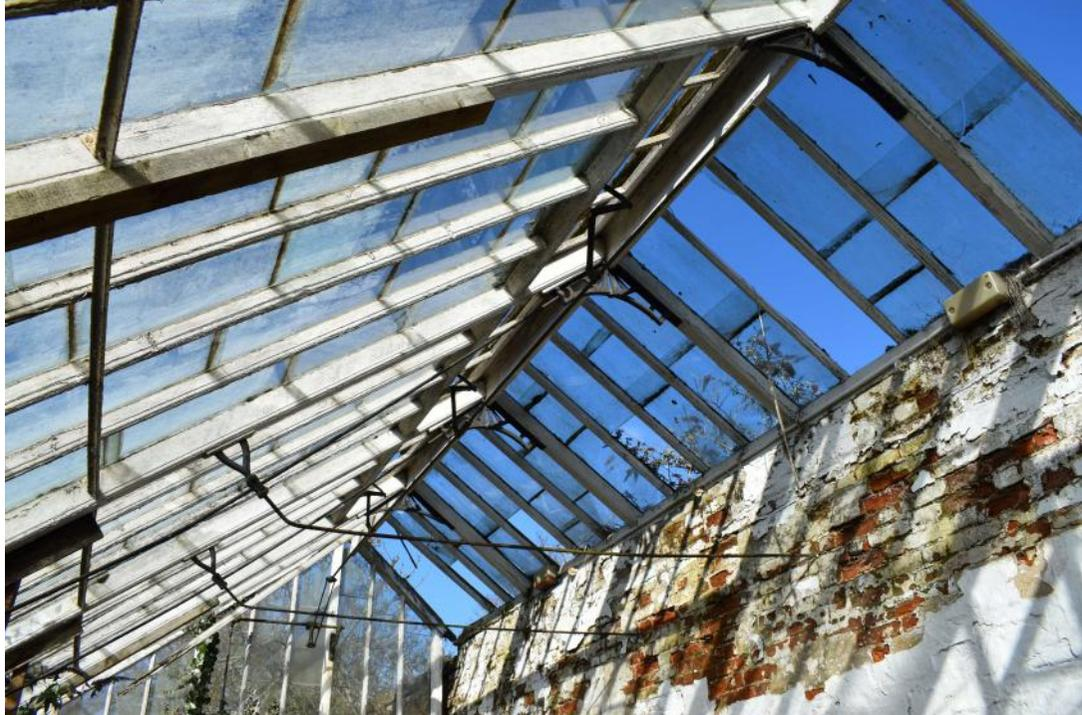
STOWG23\_Photograph\_066Detail of cast iron eave spandrels in glasshouse. Photograph taken facin...
