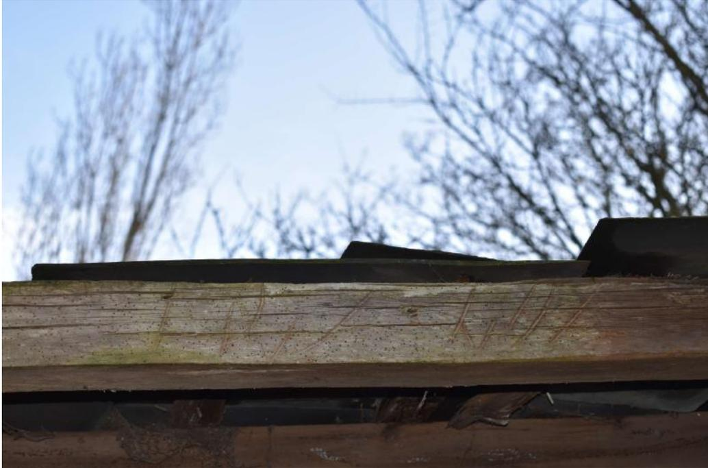
**Photograph 8** Detail of Baltic timber mark on rafter of bothy.
