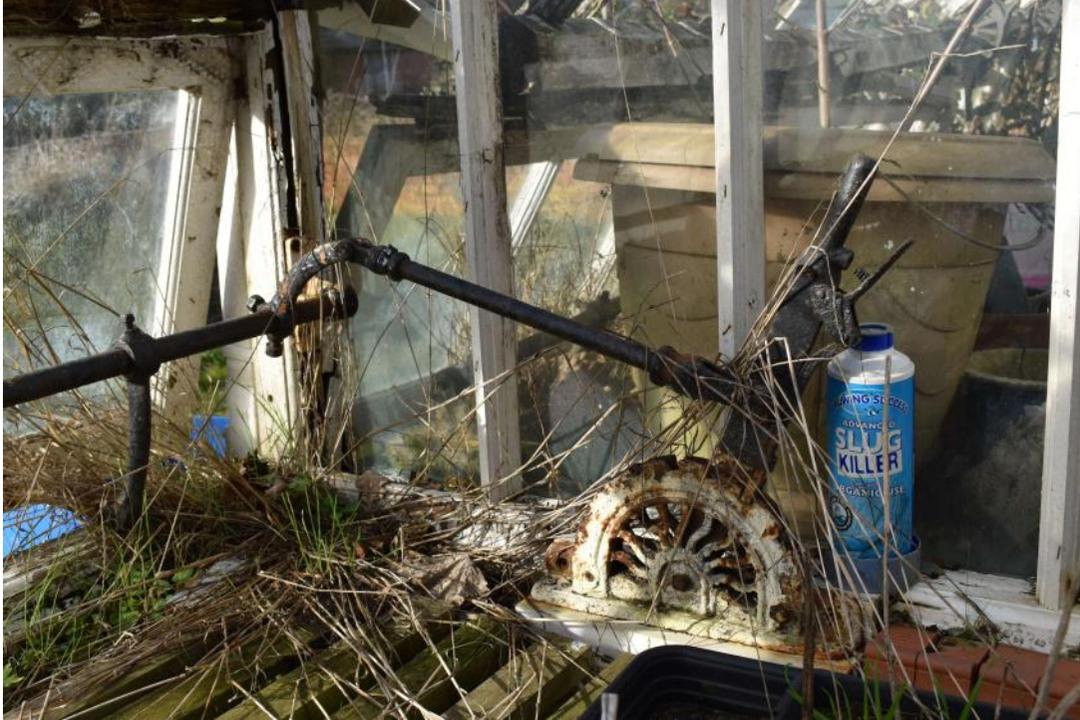
STOWG23 Photograph\_078Detail of cast iron eaves spandrels and wrought iron lower window openi...
