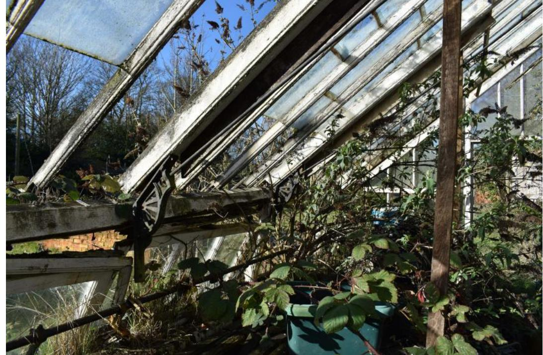
STOWG23\_Photograph\_067Detail of cast and wrought iron lower window opening/closing mechanis...
