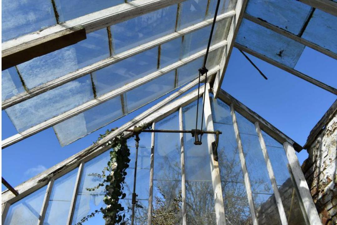
STOWG23\_Photograph\_070Detail of wrought iron lower window closing mechanism in glass...
