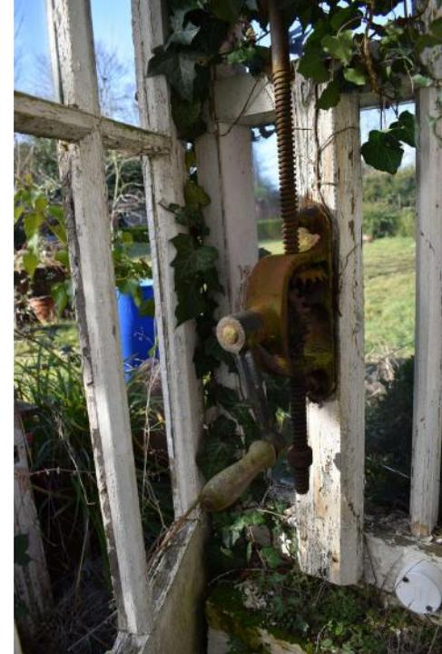
STOWG23\_Photograph\_069Detail of wrought iron upper window opening/closing mechanism in glas...
