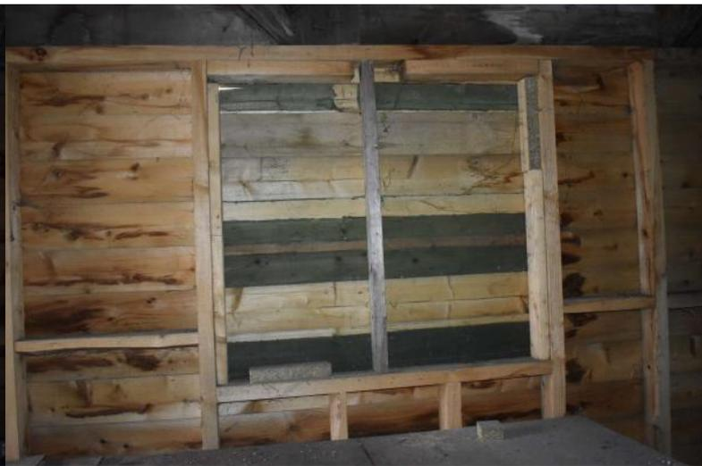
CFTF22\_PhotoGraph\_035Detail of re-used railway sleepers in eastern ... CFTF22\_PhotoGraph\_036Western elevation of store 1. Photograph ta...
