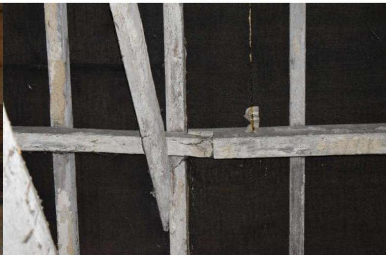
CFTF22\_PhotoGraph\_073Detail of scarf-joint in purlin on the northern ... CFTF22\_PhotoGraph\_074Detail of cut tie-beam and later timbers and ...
