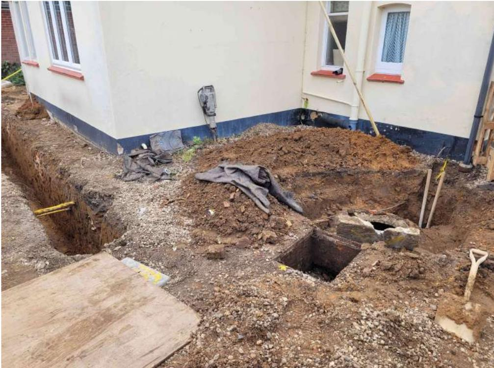
**Photograph 9** General site shot showing well in relation to manhole inspection chambers and extent of existing house, looking south-east
