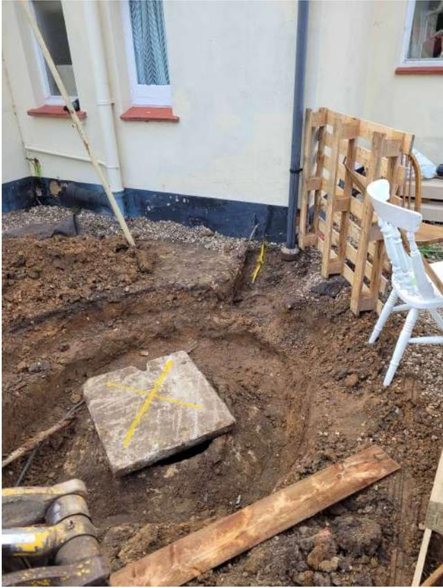
**Photograph 6** Partially exposed top of well in relation to existing property
