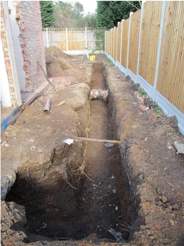
**Photograph 2** Foundation trenching to the rear/side of the property, looking north
