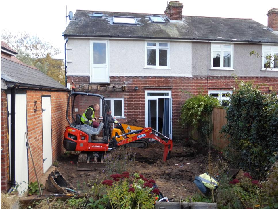
**Photograph 1:** Excavation of extension footings, looking east.
