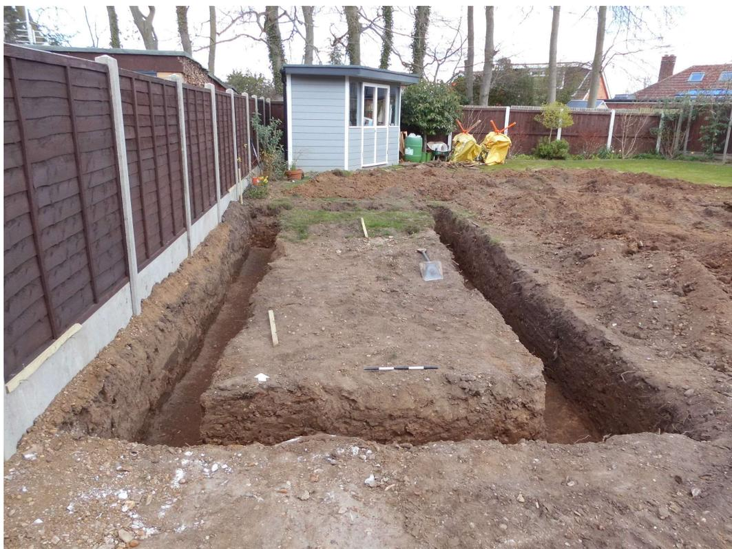
**Photograph 2** The garage foundations, looking north
