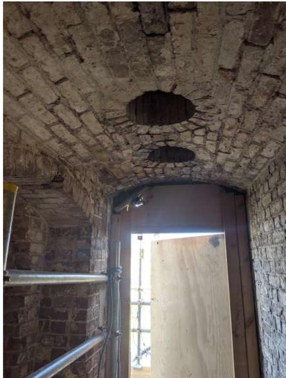
**Photograph 7** Martello Tower internal view, first-floor. Detail of smoke vents. Photograph taken facing north-west.
