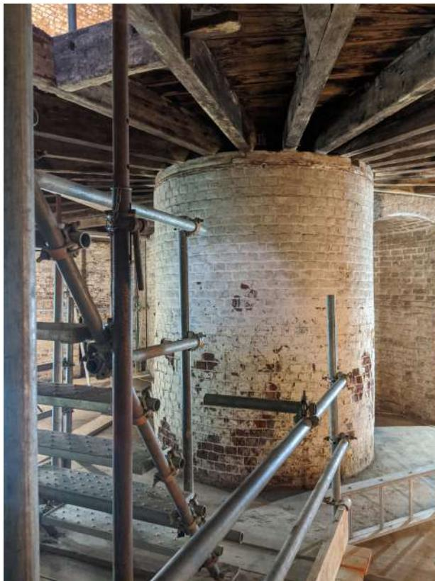
**Photograph 5** Martello Tower internal view, ground-floor. Detail of central pillar. Photograph taken facing south-east.
