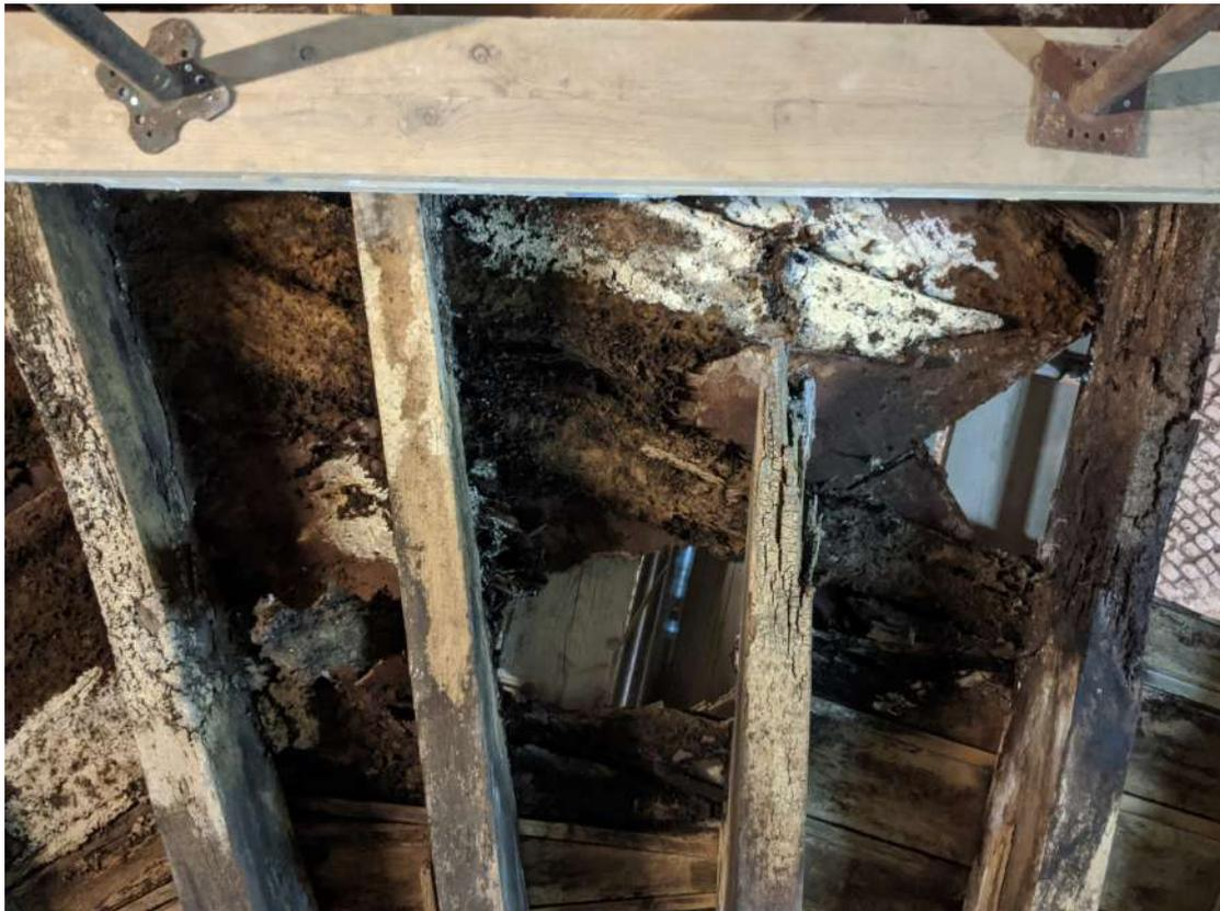
**Photograph 12** Martello Tower internal view, ground-floor. Detail of damage to floor above.
