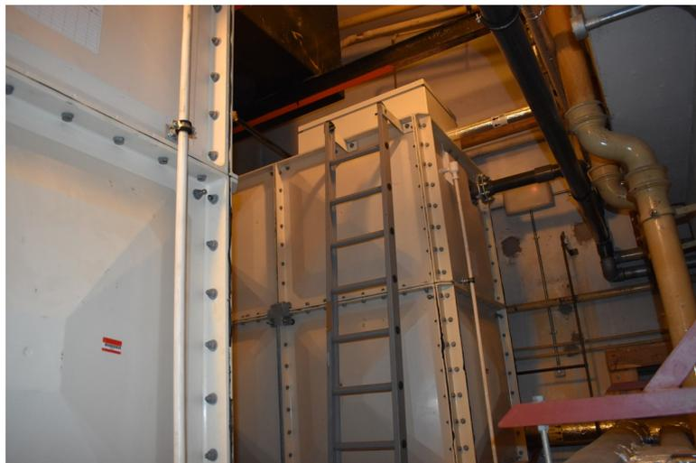
**Photograph 25** Large water tanks in roof of tower block.
