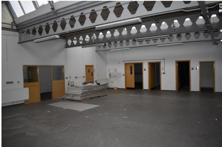
**Photograph 17** Interior of art block, showing metal beams supporting roof and sun-lights. Photograph taken facing north-east.
