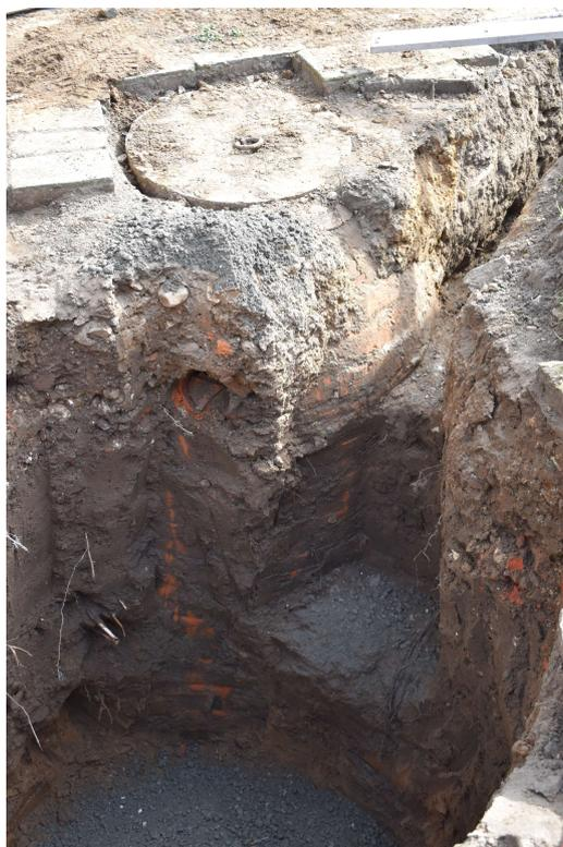
**Photograph 1** Brick soakaway F1 in the southeastern edge of the waste tank pit – looking southeast
