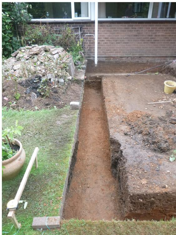
**Photograph 1** Rear extension foundation trench, looking NNE
