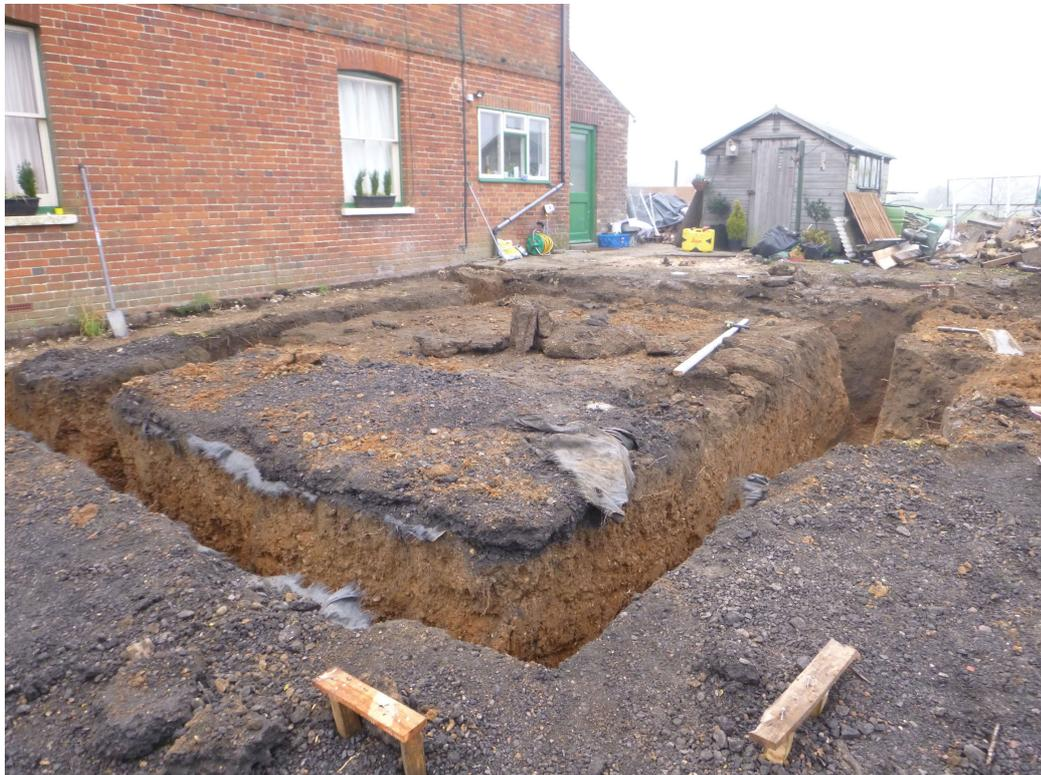
**Photograph 1** Extension: foundation trenches fully excavated, looking SW
