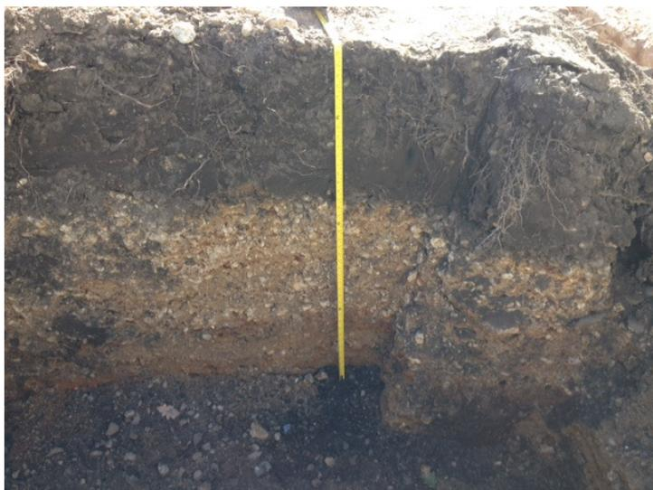
**Photograph 5** Section through road surface F1
