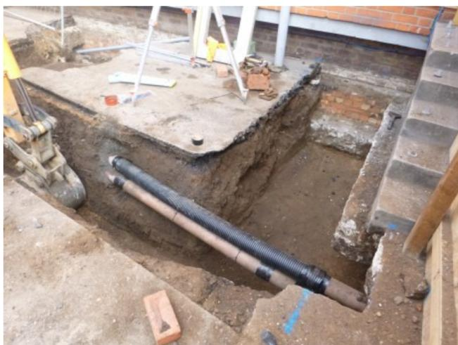
**Photograph 8** Foundation trenches for gym extension
