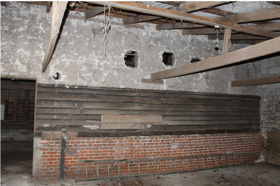
**Plate 2** Detail of the brick plinth to the Grain Barn with weatherboard above this and then render covering the upper portion of the frame – view west.
