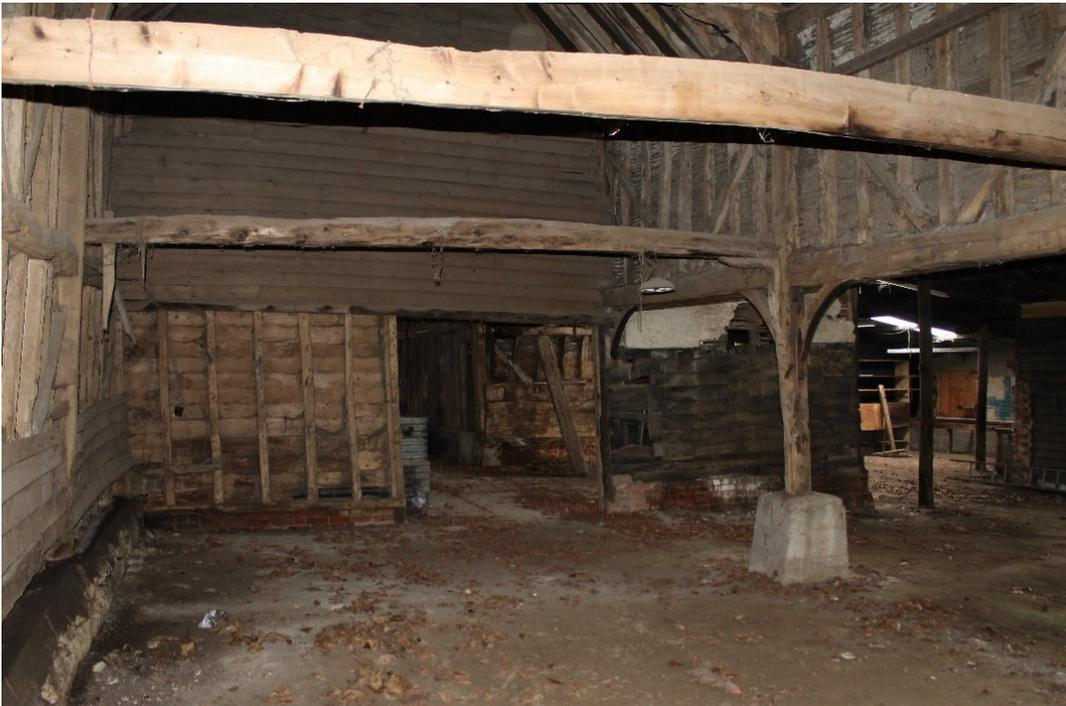
**Plate 10** The interior of bays 2-3 in the Church Barn, converted to a cart lodge by the removal of the lower framing – view east
