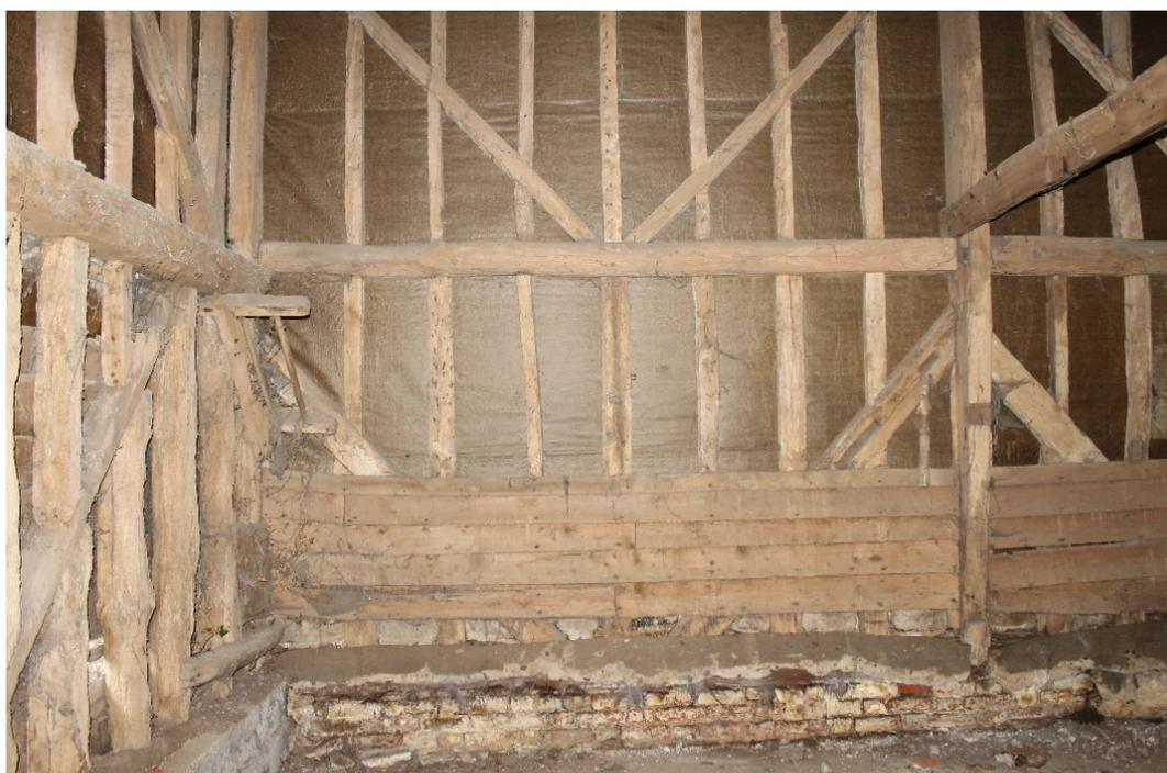
**Plate 14** Plank cladding to wall of bay 1 and remains of hay rack, indicating bays 1-3 of the Church Barn were once used to house animals - view north-west
