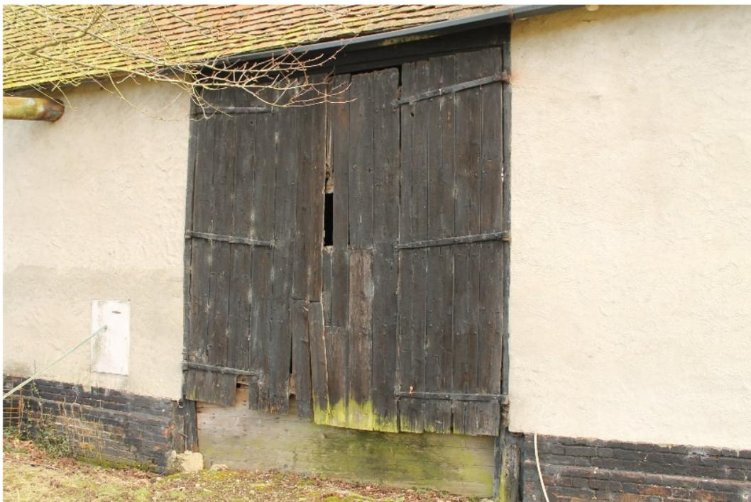
**Plate 3** Full-height barn doors in the south-west elevation of the Grain Barn with original strap and pintel hinges - view north
