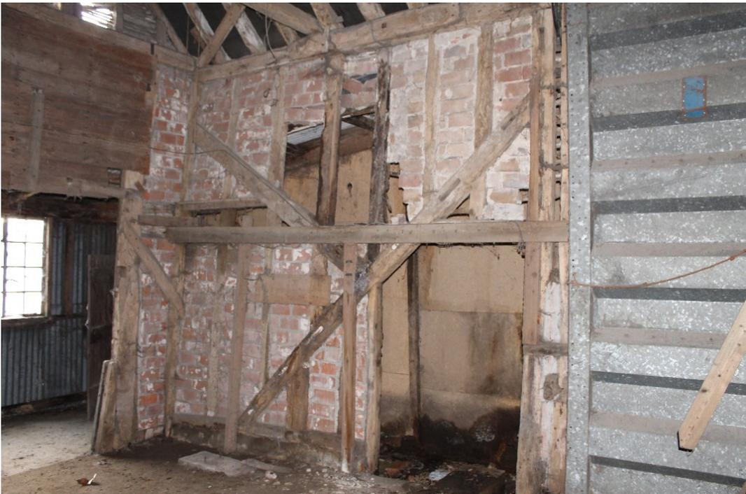
**Plate 6** South-east wall of the Grain Barn midstre showing the Y-shaped bracing and brick noggin - view east
