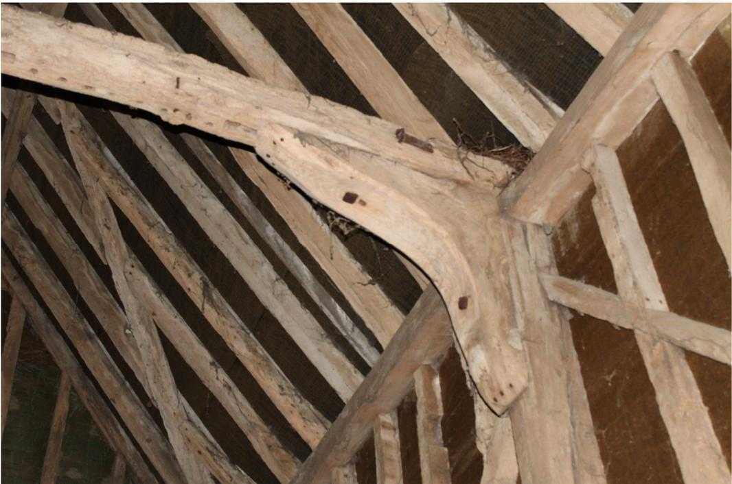
**Plate 12** Large hewn knee brace supporting re-used tie beam of truss A in the Church Barn - view west
