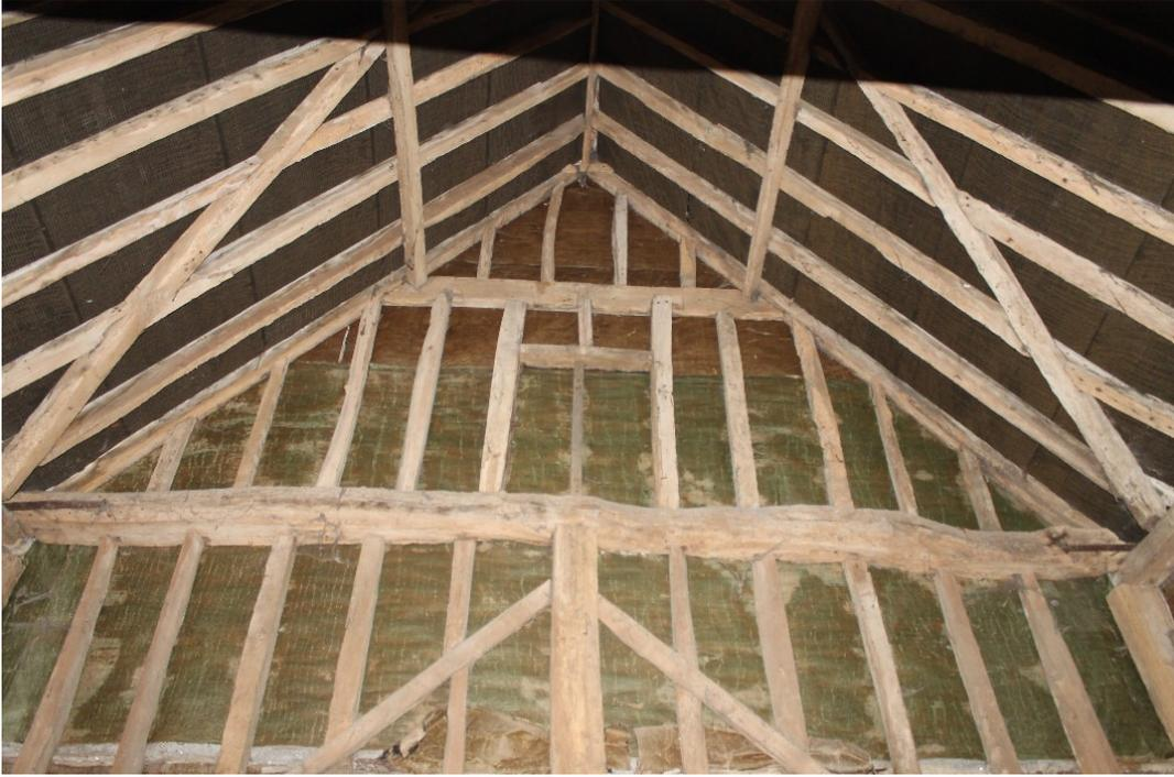
**Plate 11** South-west gable frame of the Church Barn with inserted window above the wall plate – view south-west
