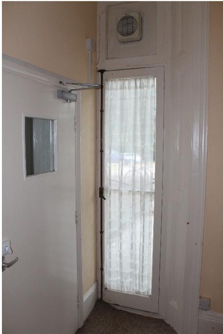
**Plate 5 Original French doors of Spurrier's House truncated by inserted stud wall - view north-west**
