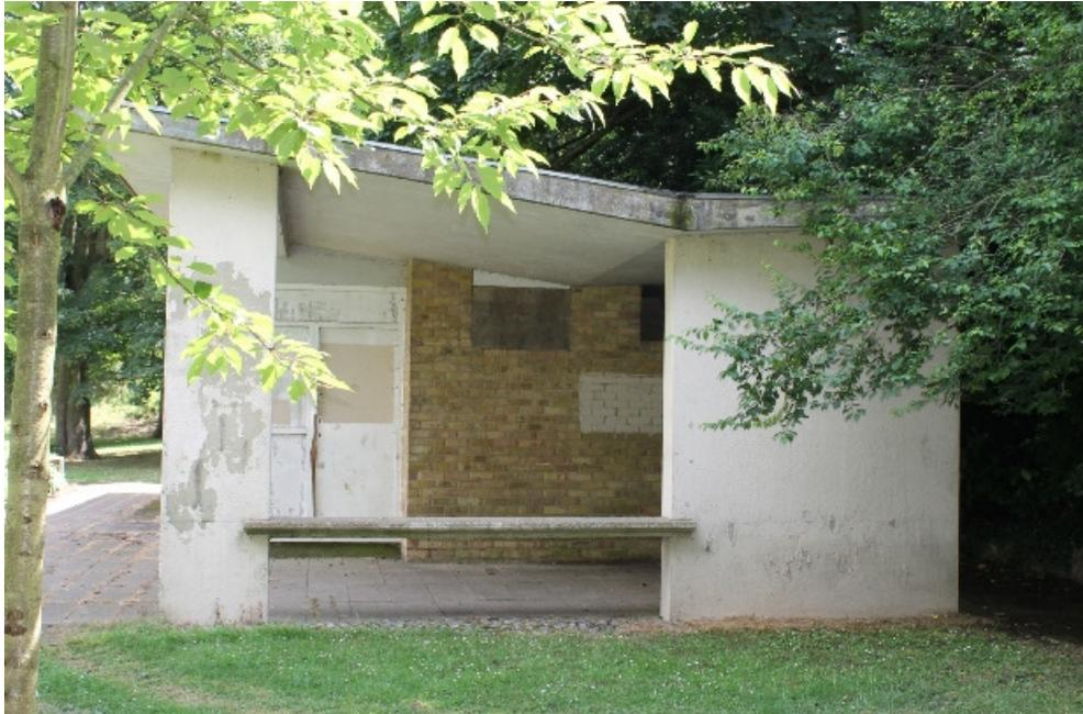
**Plate 36** The west end of the Greyhound toilets with the canopy over the bench held by the roof piers - view east
