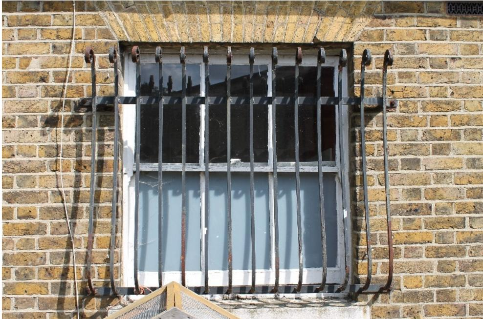
**Plate 3 Detail of wrought iron security bars on extension to Spurrier's House
