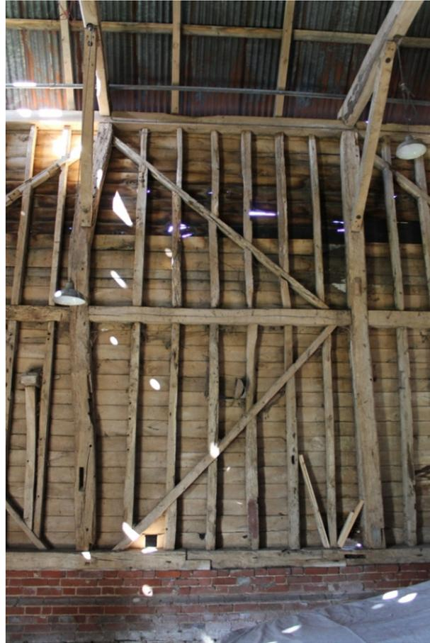
**Plate 7** Framing of bay 6, showing the primary bracing forming a diamond pattern - view north-west
