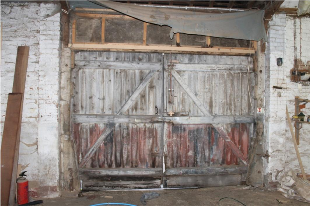
**Plate 9** Bay 2 of the brick barn, showing later cart doors attached to original doorposts, sawn from single timbers and incorporating flared bases - view north-east.
