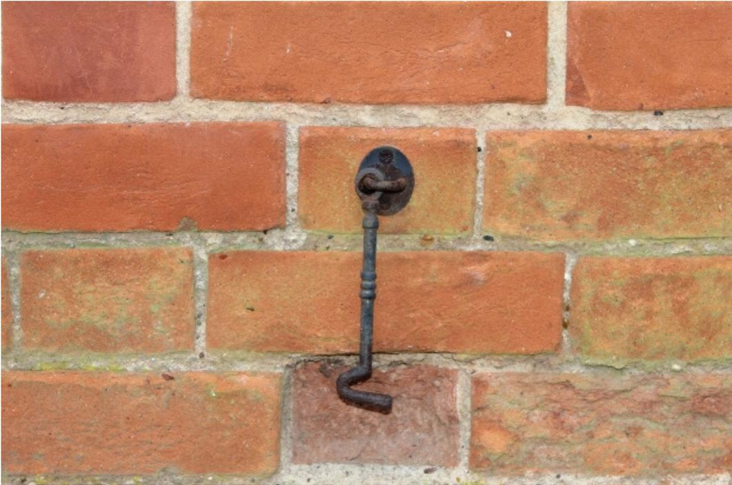
**Plate 3** Hook for holding open cart doors on north-west elevation – view south-west
