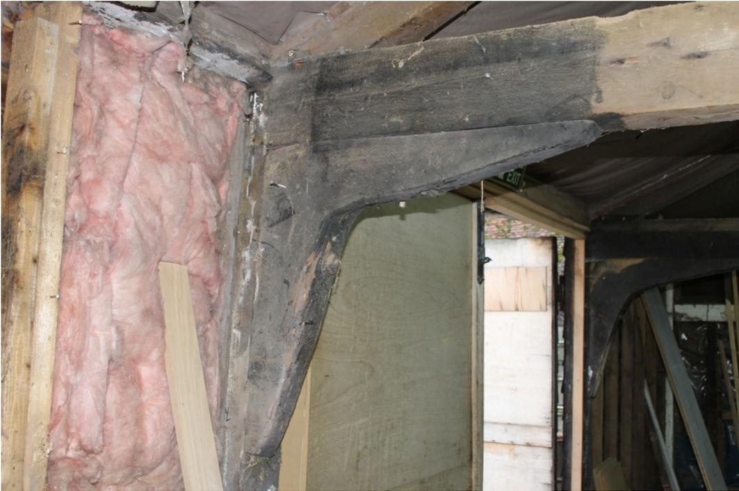
**Plate 15** Knee brace to south-east post of truss A, with tie beam carried on the head of the post and the wall plate supported by the tie beam - view east
