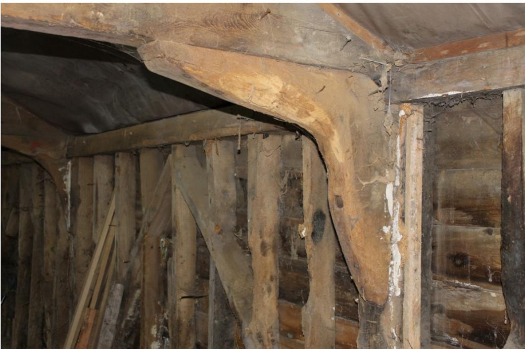
**Plate 14** Knee brace to north-west post of truss A, with tie beam sitting on top of wall plate - view south-west
