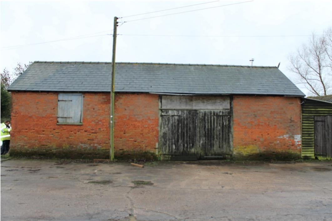
**Plate 1** Brick barn at Betts Farm, north-east elevation, with ?original pitching door and later cart doors - view south-west
