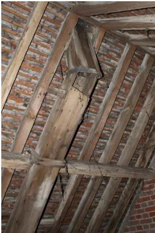
**Plate 28** Structure 1/2, showing one of the original timber-cased ventilation shafts rising through the building and exiting the attic roof – view south-east
