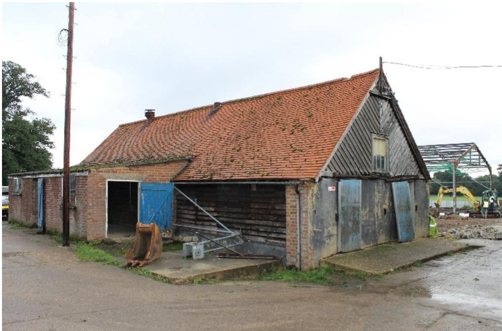
**Plate 88** Structure 10 milking shed with post-1956 lean-to and sliding doors to south elevation - view north-east
