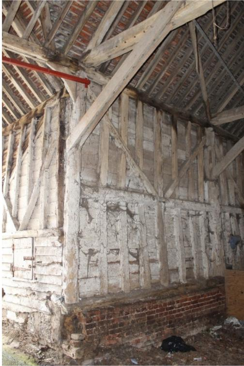
**Plate 83** Structure 6 barn, north-east post to truss D with jointed straight brace and additional straight bracing nailed to the face of post and tie beam – view east
