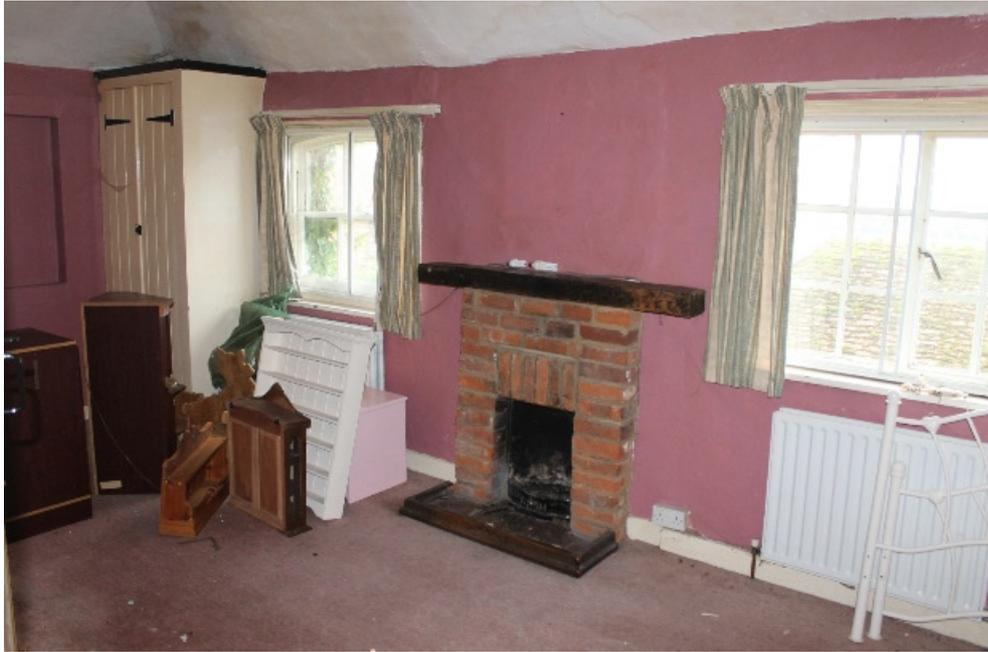
**Plate 37** Structure 1/2, interior of Garage Flat sitting room, showing the fireplace to the inserted chimney stack and the blind openings converted to windows on either side. The sash window to the left of the fireplace has been relocated from the opening visible on the extreme left of the photograph – view north-east
