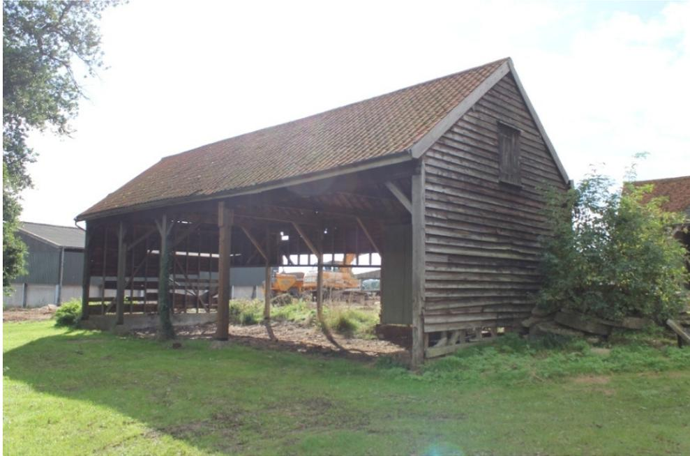
**Plate 65** Structure 5 Dutch barn, showing the open-fronted north-east elevation with the two missing truss posts and the pitching door of the north-west elevation - view south-east
