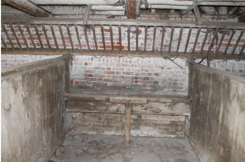
**Plate 53** Structure 4 cow house, interior of stall 3 showing the manger with tethering ring and hay rack above - view north-east
