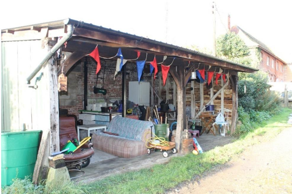
**Plate 104** Structure 22 tool shed opposite Farm Cottage, built up against the wall of the laundry drying ground and showing the lightly arched braces to the posts and the low brick plinths and sill beams supporting the posts – view west
