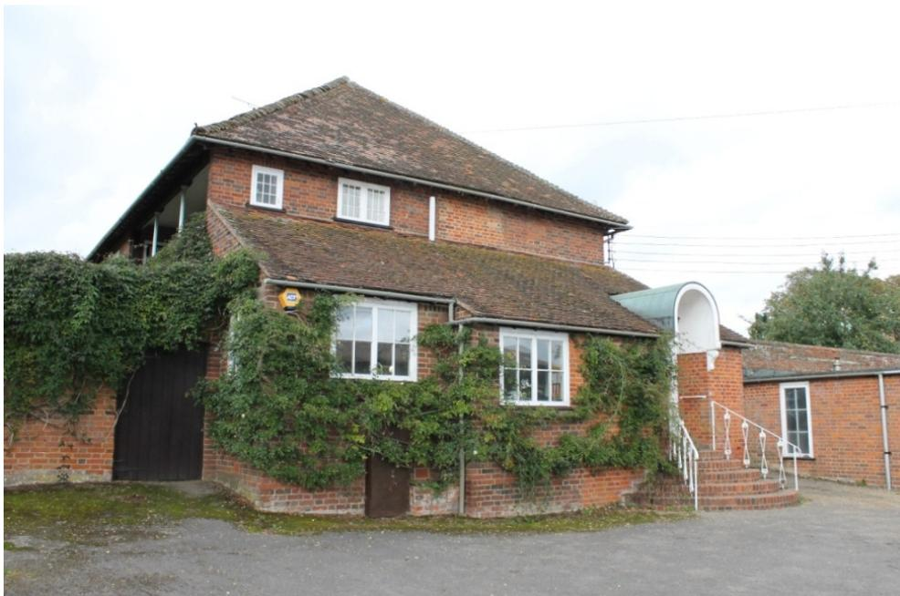
**Plate 120** Structure 17 Garden House west elevation showing the single-storey extension with attenuated door hood and the recessed veranda on the first floor – view north-west
