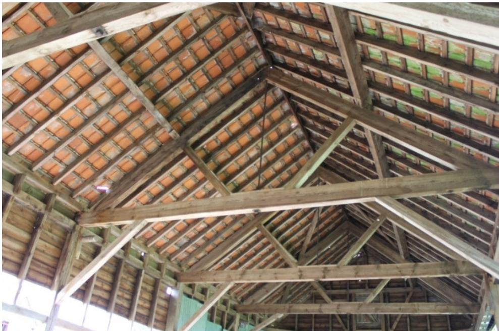
**Plate 66** Structure 5 interior of the Dutch barn, showing the king bolt roof trusses - view east
