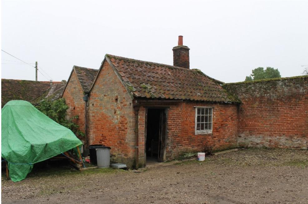
**Plate 43** Structure 3a the gardener's stores, showing the gabled ends of the western bays and the inserted sash window in the north-west elevation - view south-east
