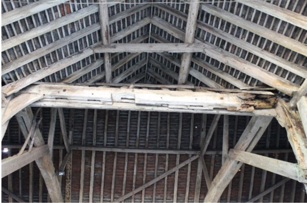
**Plate 77** Structure 6 barn, wall plate to north-east side of bay 2 with exposed mortices which indicates the midstrey is a later addition - view south-west
