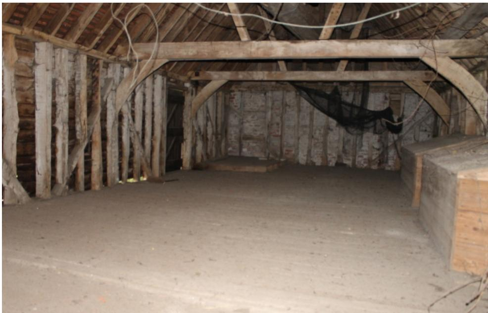
**Plate 56** Structure 4 interior of granary showing raised platform around the granary access and the inserted pitching door of the south-west frame - view north-west
