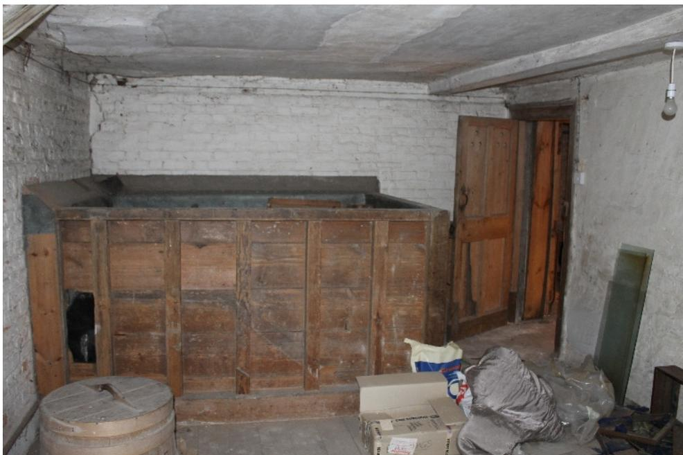
**Plate 20** Structure 1/2, interior of FF2 showing the 19th-century grain bin delivering grain to stable 1 below - view south-east
