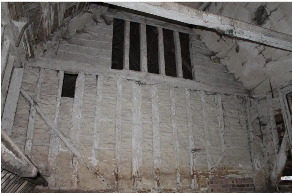
**Plate 50** Structure 4 granary/cow house, north-west elevation concealed by the 19th-century infill building showing the exposed timber frame and the brick noggin - view south-east
