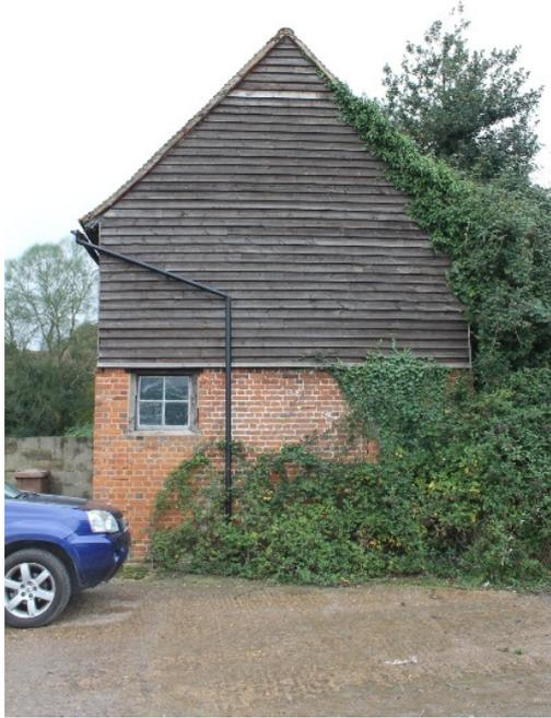
**Plate 49** Structure 4, granary/cow house, south-east elevation showing the inserted window above the rebuilt corner - view north-west
