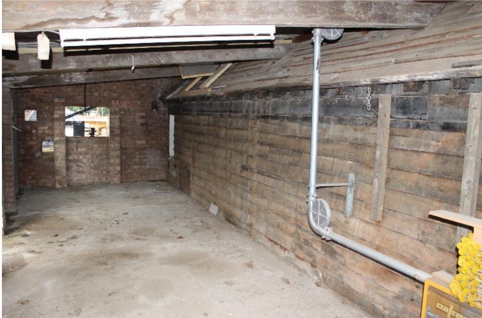
**Plate 89** Structure 10 original weather-boarding to the earlier timber-framed building, concealed by the post-1956 lean-to. The ventilation hatches extending the length of the building can be seen below the eaves – view north-east
