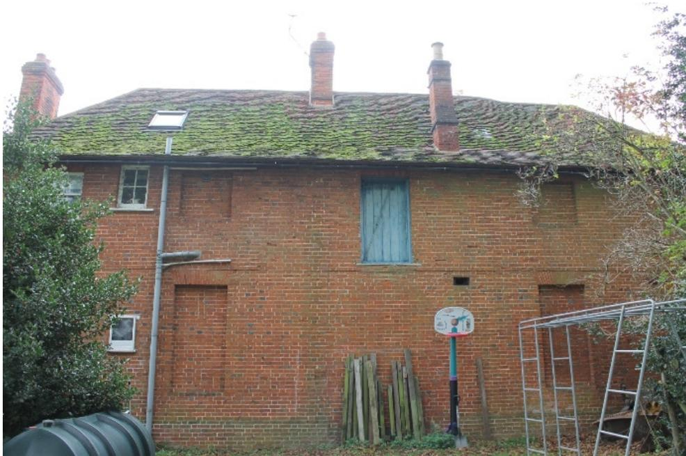
**Plate 9** Structure 1/2, the north-east elevation of the north range, originally with blind windows to both ground and first floor. Windows have been inserted for Stable Cottage on the left and a doorway with a grain hoist has been inserted in the central window of the first floor. Below this there appears to be a blocked double doorway - view south-west
