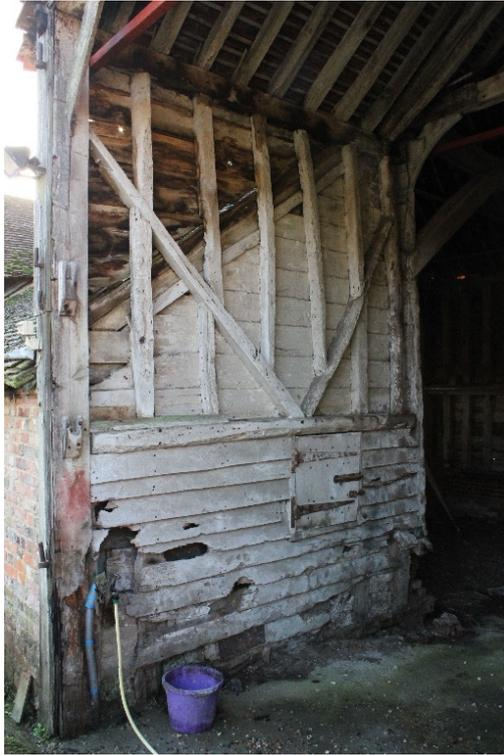
**Plate 85** Structure 6 barn, west midstrey with weatherboard to lower register and inserted hatch to lean-to 2 – view south-east
