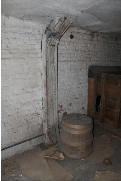
**Plate 21** Structure 1/2, interior of FF2 showing the 18th-century timber-cased ventilation system rising from stable 1 below - view north-east
