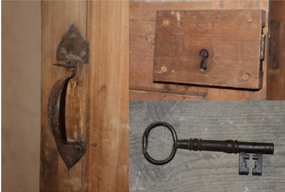
**Plate 19** Structure 1/2, detail of original door latch, lock casing and door key re-used on the 19th-century four panel doors to the grooms' rooms on the first floor of the main range
