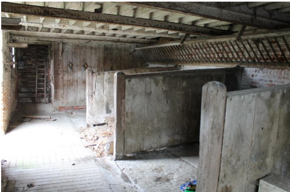
**Plate 52** Structure 4 interior of cow house, with the stalls to the right and the grain box to the rear. The inserted I-beams can be seen below the granary floor joists and the ladder to the granary is in front of the blocked doorway to the infill building on the left - view north-west
