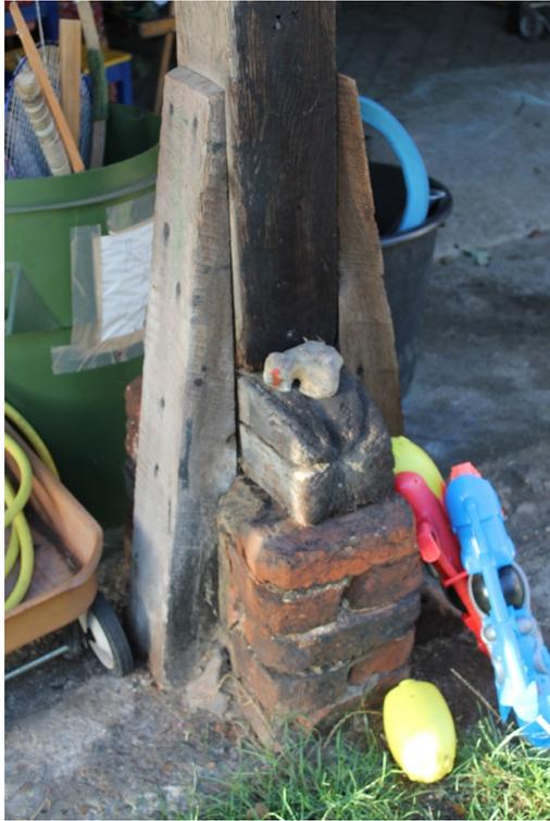
**Plate 105** Structure 22, detail of the low brick plinth and sill beam supporting the central post – view south-west
