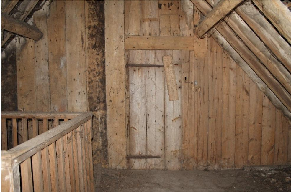
**Plate 25** Structure 1/2, attic landing showing the inserted timber dividing wall between the attics of the main range and Stable Cottage, with the Georgian staircase to the left - view south-east
