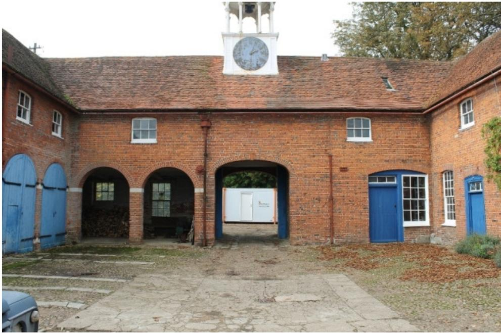
**Plate 5** Structure 1/2, the south-east elevation of the main range of the stable block with the inserted entrance to stable 1 to the right of the carriage arch and the inserted arches to garage 1 on the left of the carriage arch. The coach house with Garage Flat above is to the left whilst the tack room is on the right - view north-west
