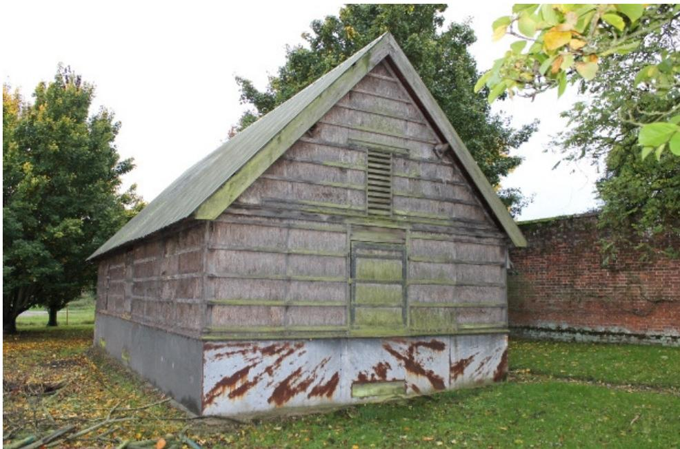
**Plate 100** Structure 20 north-east elevation of the apple store showing the rodent-proof metal skirt and the timber and straw insulating layer applied to the building – view south-west
