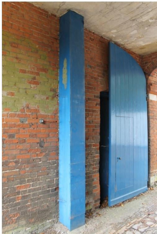
**Plate 4** Structure 1/2, interior of the carriage arch showing one of the timber boxes housing the clock counterbalance with one of the original stable doors behind the blue gate - view west
