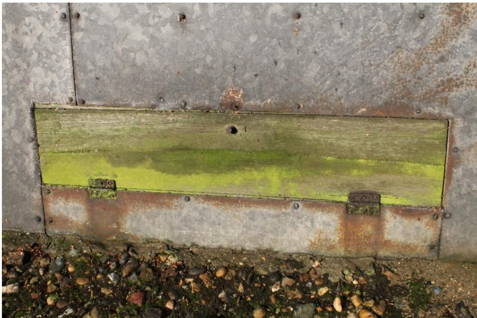
**Plate 101** Structure 20 apple store, detail of the hinged ventilation hatch in the metal skirt
