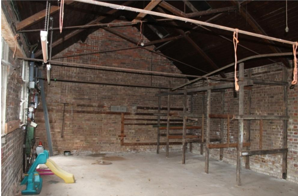
**Plate 97** Structure 15 interior of the workshop showing the king bolt roof trusses – view west
