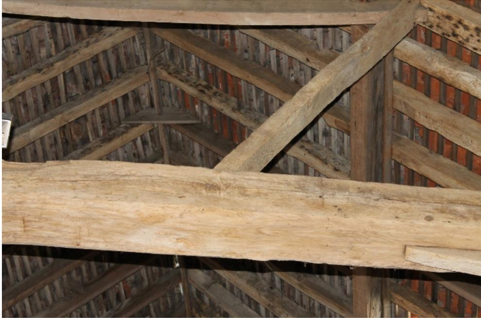
**Plate 81** Structure 6 barn, detail of tie beam, raking strut and collar on south-west side of truss A with machine-cut purlins and re-laid rafters
