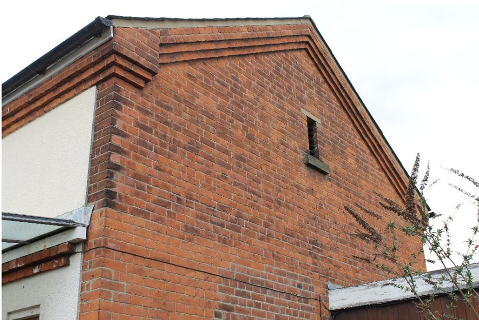
**Plate 10** East elevation of MEE 03, showing ventilation louvre in gable end - view north-west
