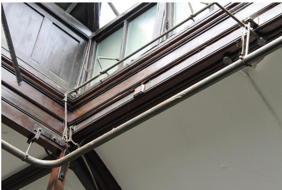
**Plate 42** HYD 08 Billiard Room, detail of the metal armatures governing the opening and closing of the lantern windows
