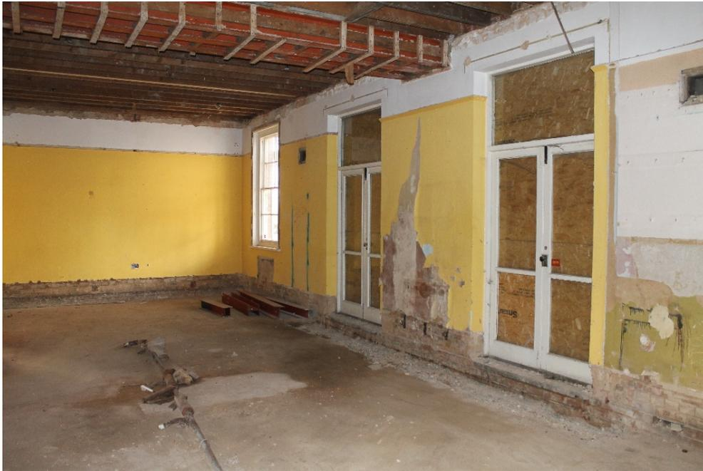
**Plate 43** HYD 08 bedrooms converted to bar, with windows altered to French doors
