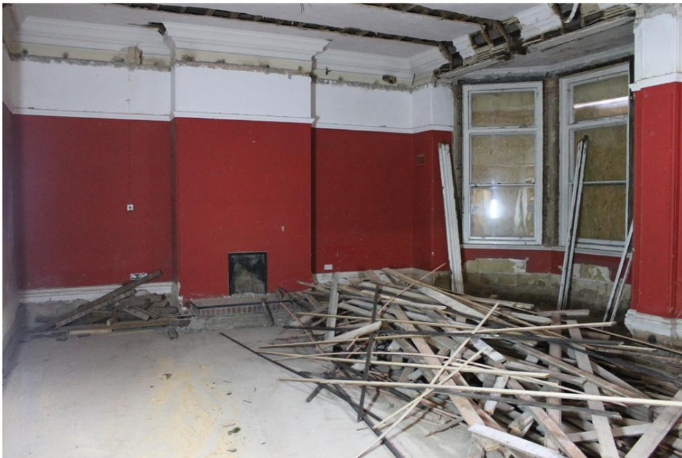
**Plate 36** HYD 08 Ante Room, showing the working fireplace and evidence for the lowered ceiling – view south
