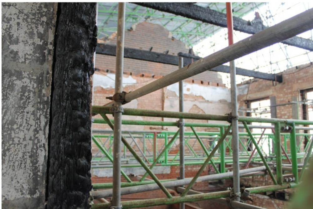
**Plate 57** Charred tie beams of HYD 11, showing evidence for king post roof trusses – view south-east
