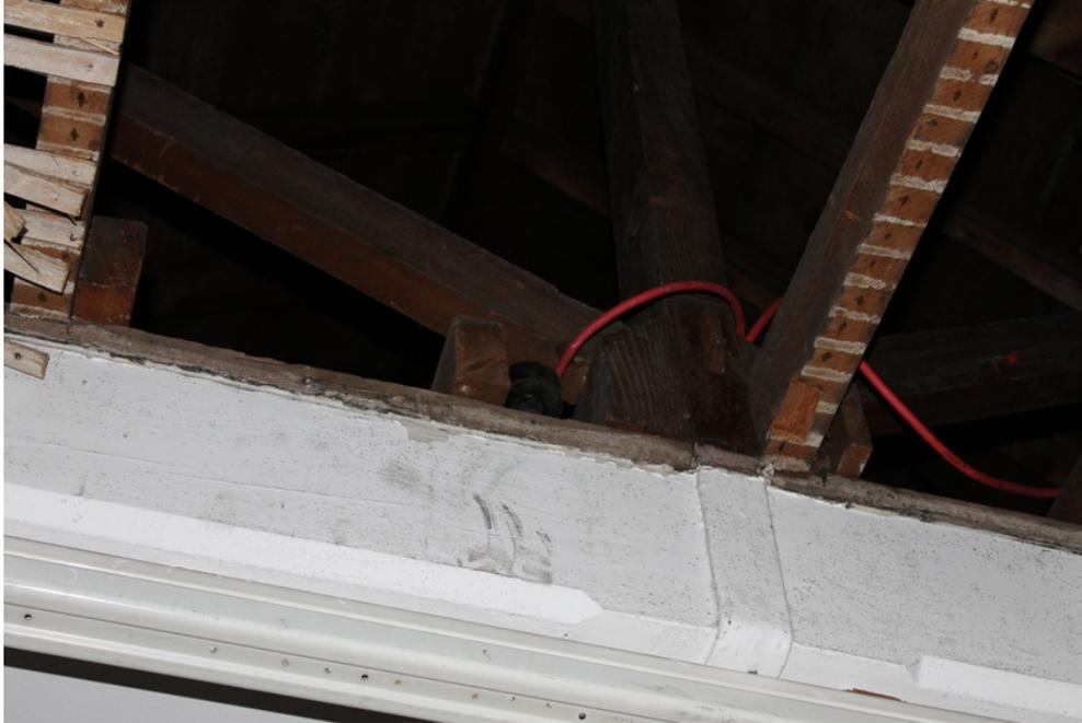
**Plate 29** Exposed king post roof truss in MEE 17
