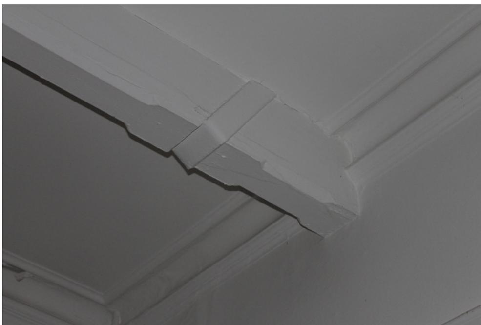
Plate 28 MEE 17 exposed chamfered tie beam of roof truss, with recess for iron strapping
