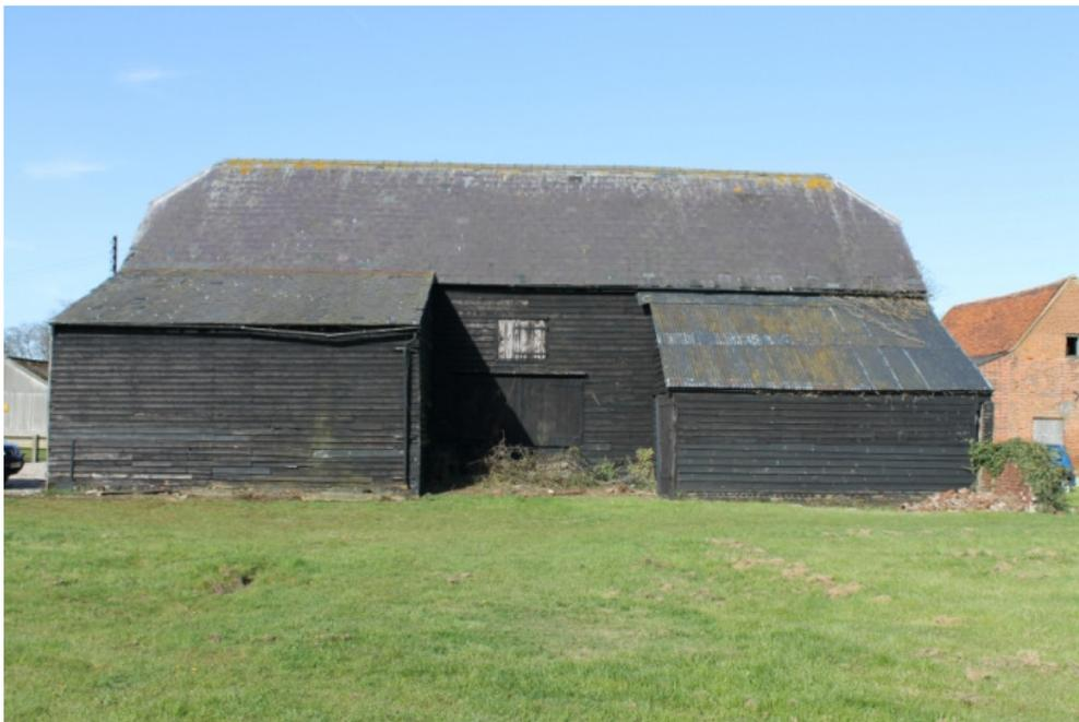
**Plate 2** North-east elevation of structure 1, showing rear barn doors and pitching door of barn 1a with lean-to 1f to the left and lean-to 1e to the right – view south-west
