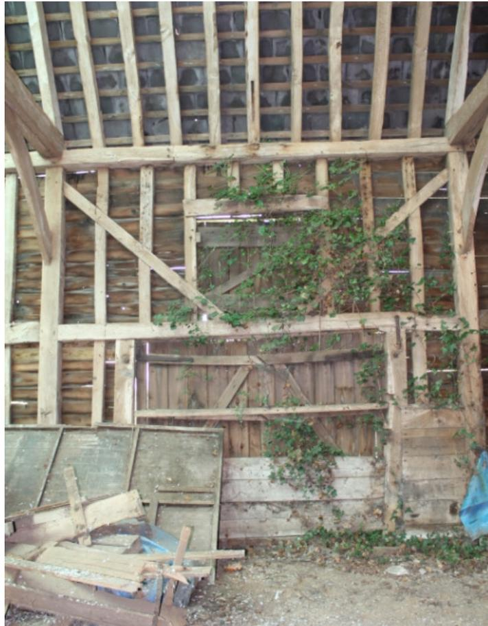
**Plate 25** Barn 3a, showing rear barn doors with replacement girding beam and threshold leap – view west
