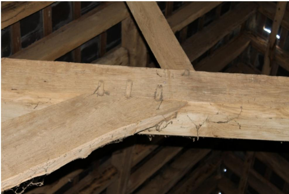
**Plate 16** Barn 2a, chiselled carpenters' marks 'III' on tie beam and strut of truss C
