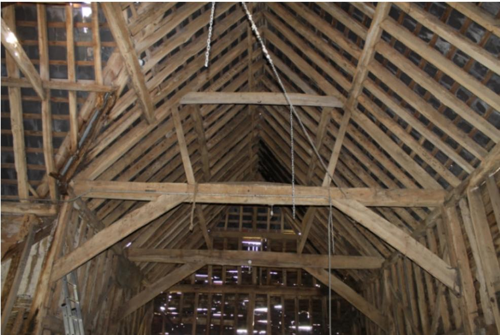
**Plate 14** Barn 2a, showing truss B with lightly curved braces, inclined queen struts and joggled purlins - view east
