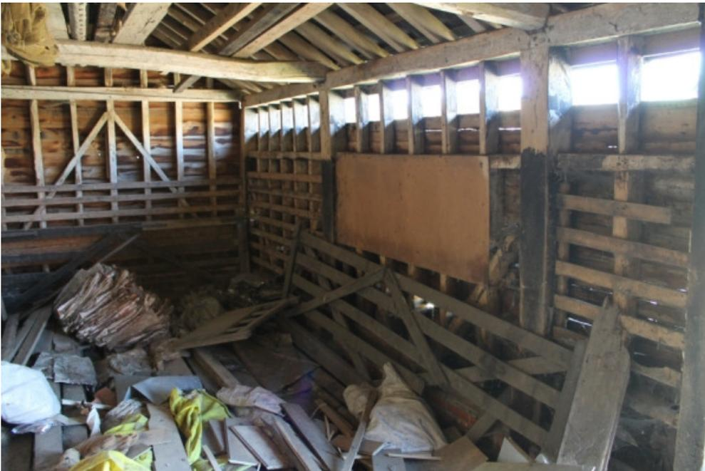
**Plate 8** Interior of lean-to 1d, showing the differences between the framing of the short end and long side – view south
