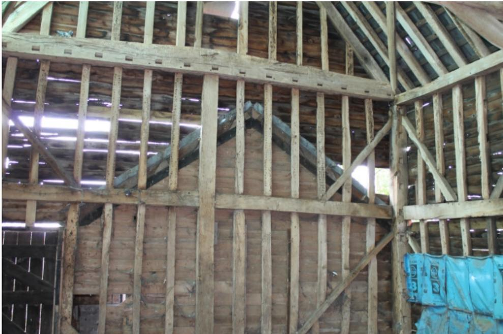
**Plate 24** Barn 3a, showing the reused tie beam in place of the wall plate – view north-west
