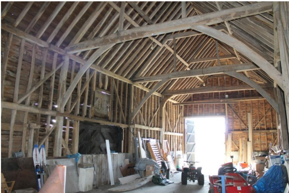
**Plate 4** Interior of barn 1a showing trusses B and C with curved bracing and queen posts and truss D with knee braces – view south-east
