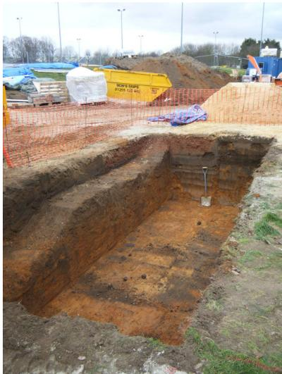
**Plate 3** The pit for a new soakaway
