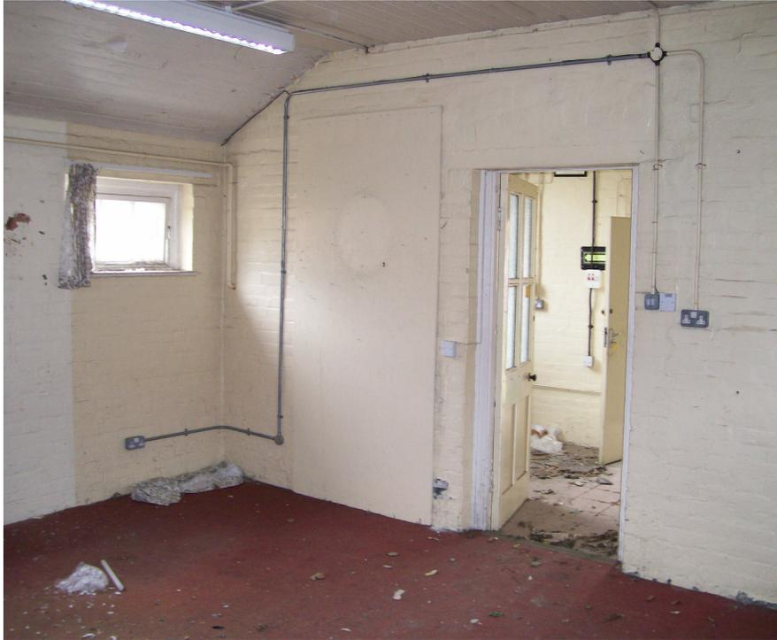
**Plate 13: Building 7; the Ablution House, showing the original tiled floor and roof and the altered doorway.**
