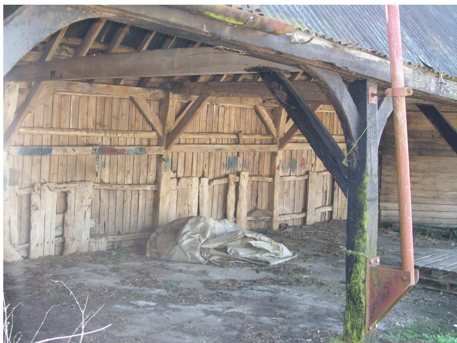
**Plate 10** Building C, interior showing three-way bracing.
