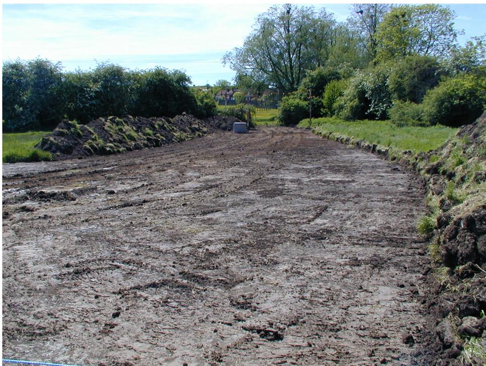
**Plate 1 Soil-stripping of the central section.**
