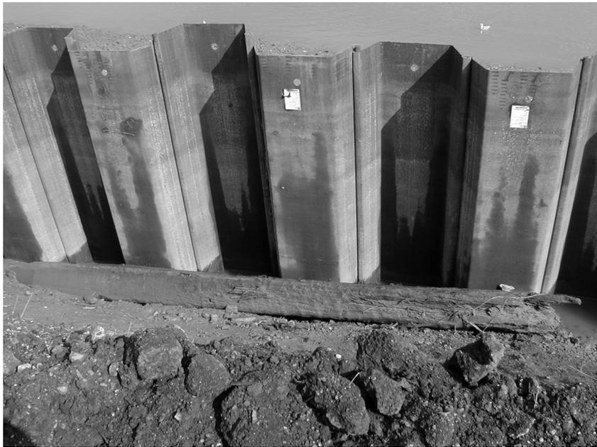
**Fig 3 Timber post with new sheet piling behind.**
